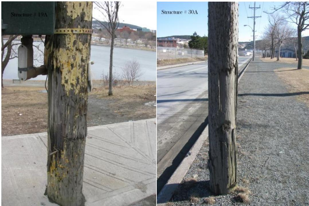
**Figure 3 – Deteriorated poles 16L**
