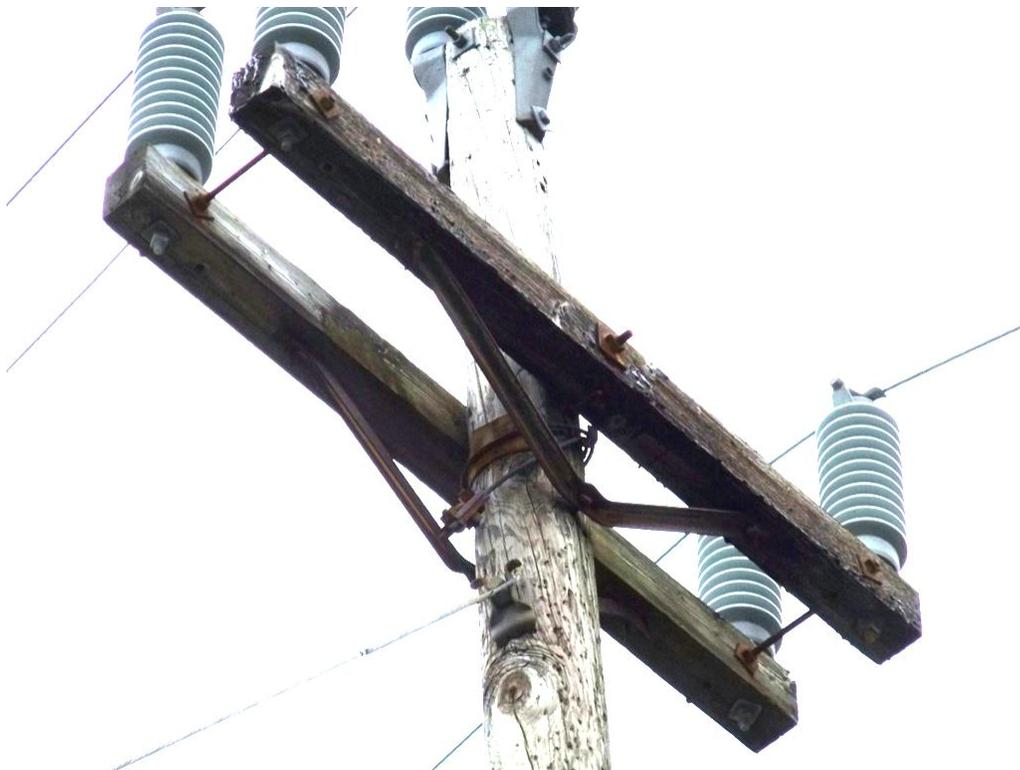
Figure 8 – 12L – Deteriorated crossarms
