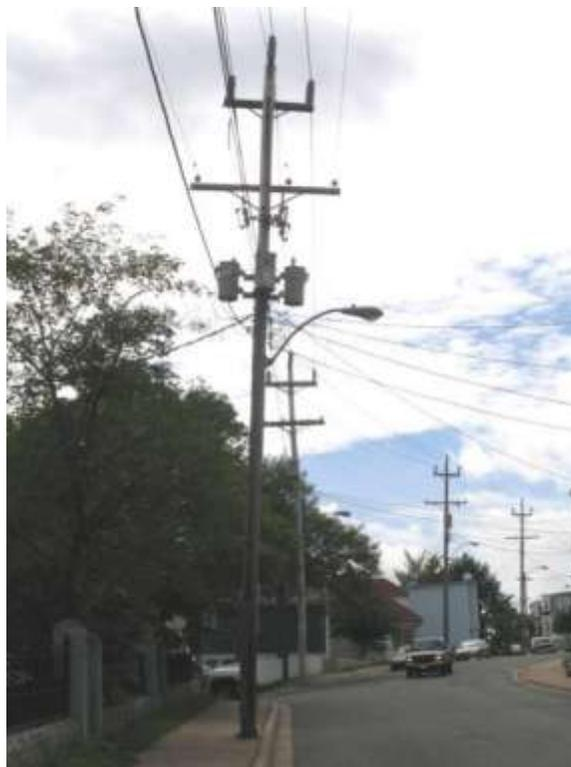
Figure 8 – 13L - Heavily loaded pole leaning
