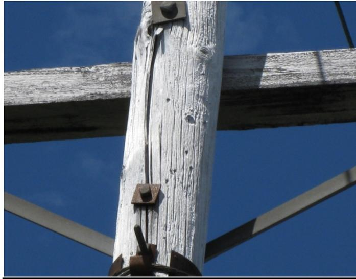
Pole Crack between Bolts
