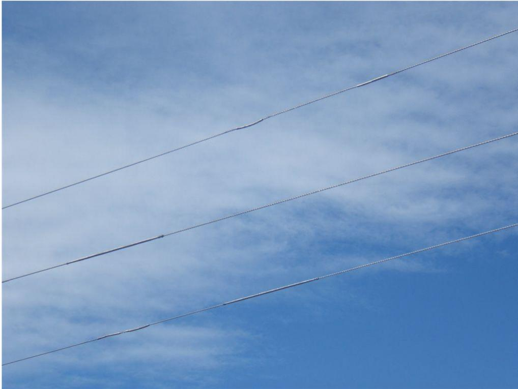
**Figure 1 – 110L – Multiple sleeves to repair conductor damage**
