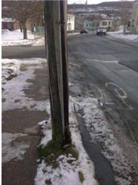
Figure 7 – 13L - Deteriorated pole showing shell separation
