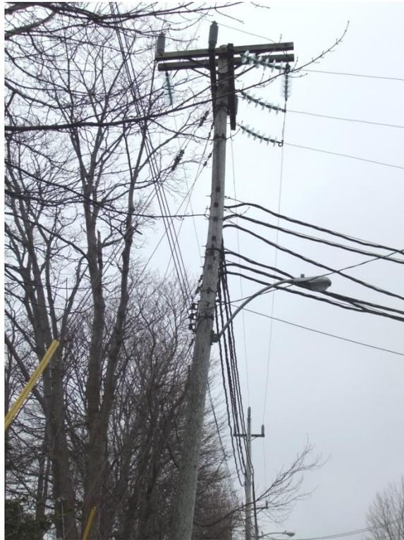
Figure 7 – 12L – Pole bent due to significant loading
