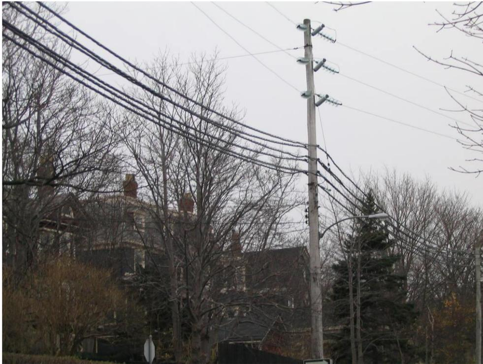
Figure 9 – 12L – Distribution aerial cable arrangement (1)
