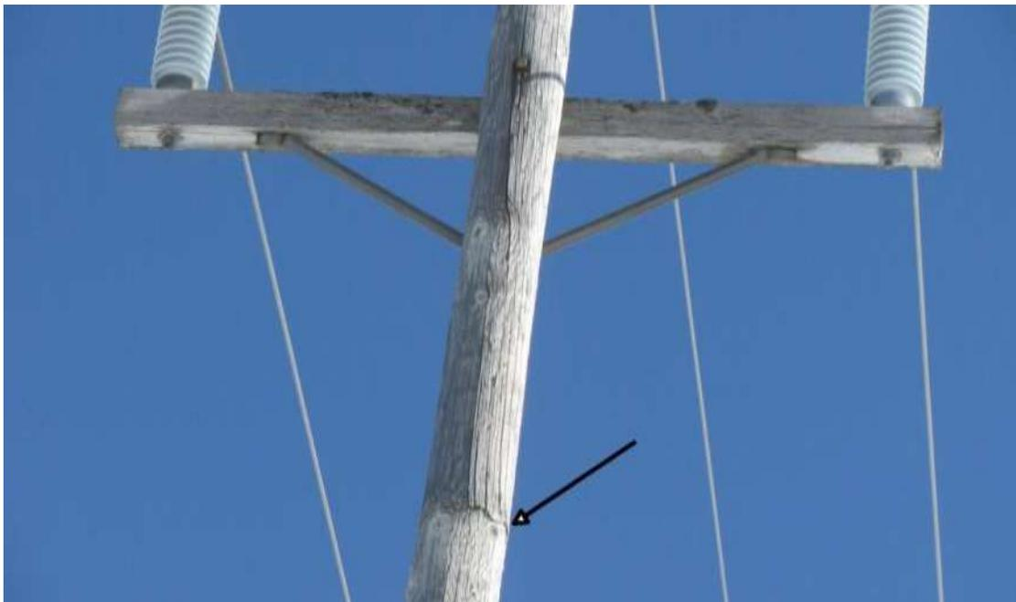
Figure 16 – 35L - Horizontal crack in pole
