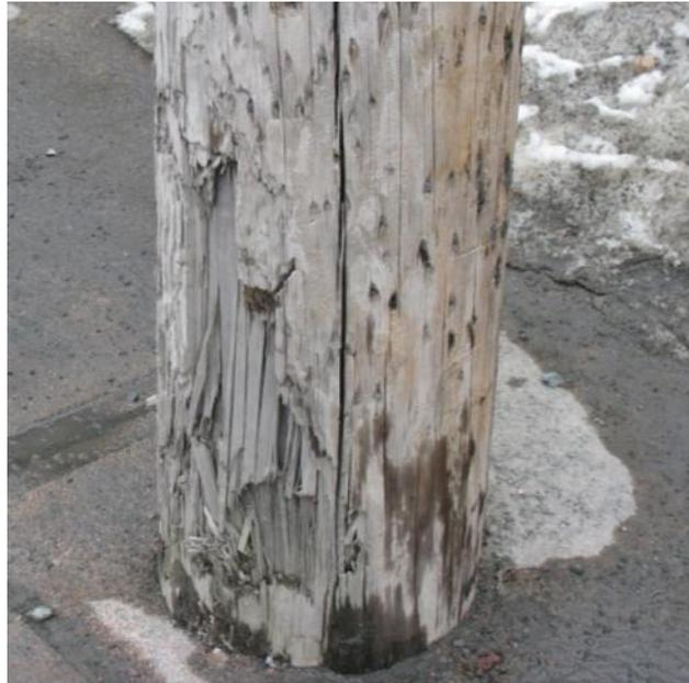
**Figure 1 – Pole damaged by vehicle 16L**
