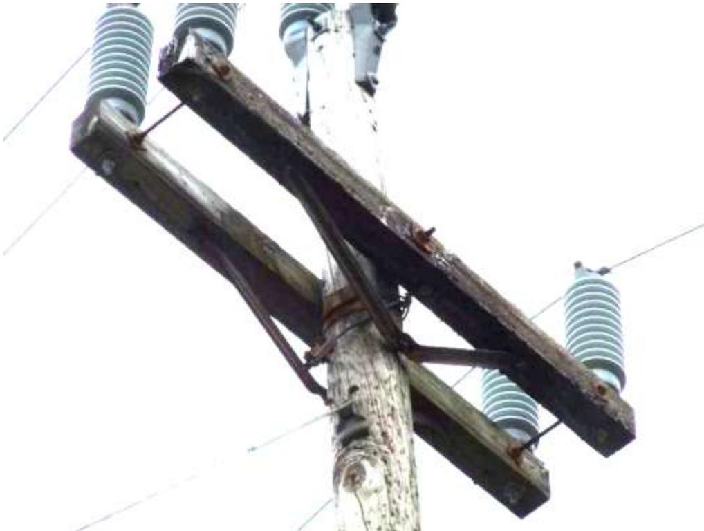
Figure 4 – 12L - Deteriorated Crossarms
