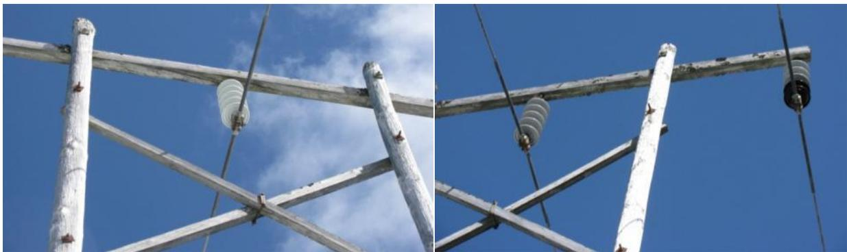
**Figure 18 – Deteriorated poles, crossarms and hardware 25L**
