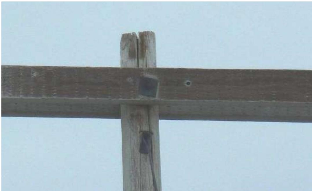
**Figure 20 – 68L - Deteriorated pole and crossarm**
