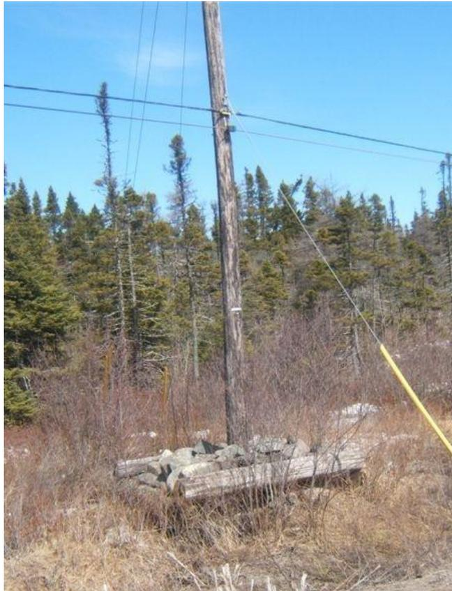
Figure 3 – 110L – Deteriorated pole and crib
