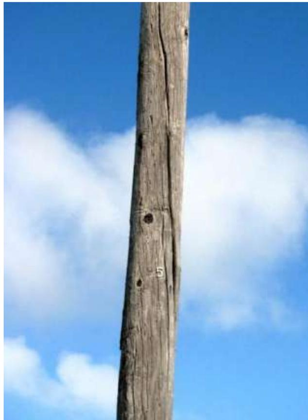
**Figure 14 – 35L - Severely deteriorated pole**
