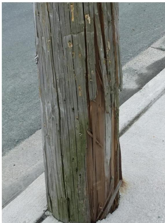
**Figure 6 – 12L – Pole showing shell separation and damage**
