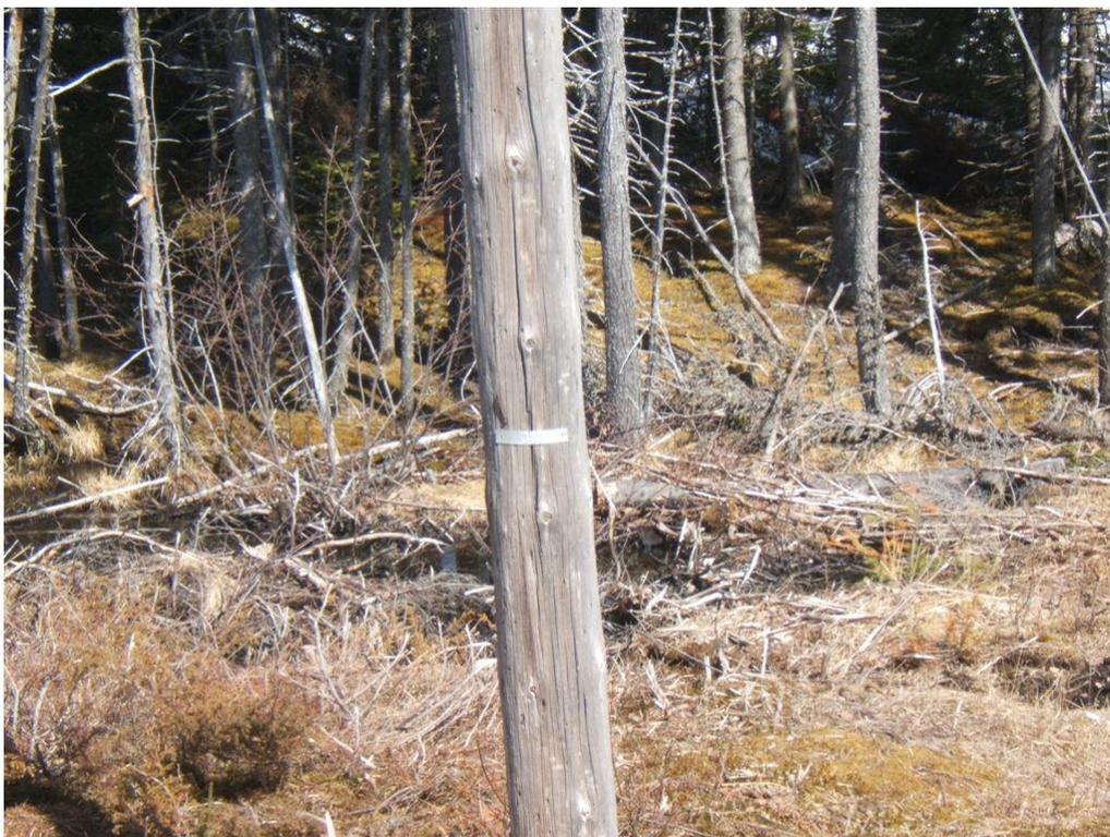
**Figure 2 – 110L – Checks in pole**
