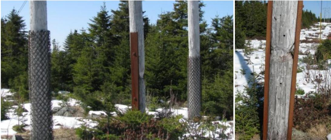
**Figure 13 – Damaged pole requiring external support 25L**
