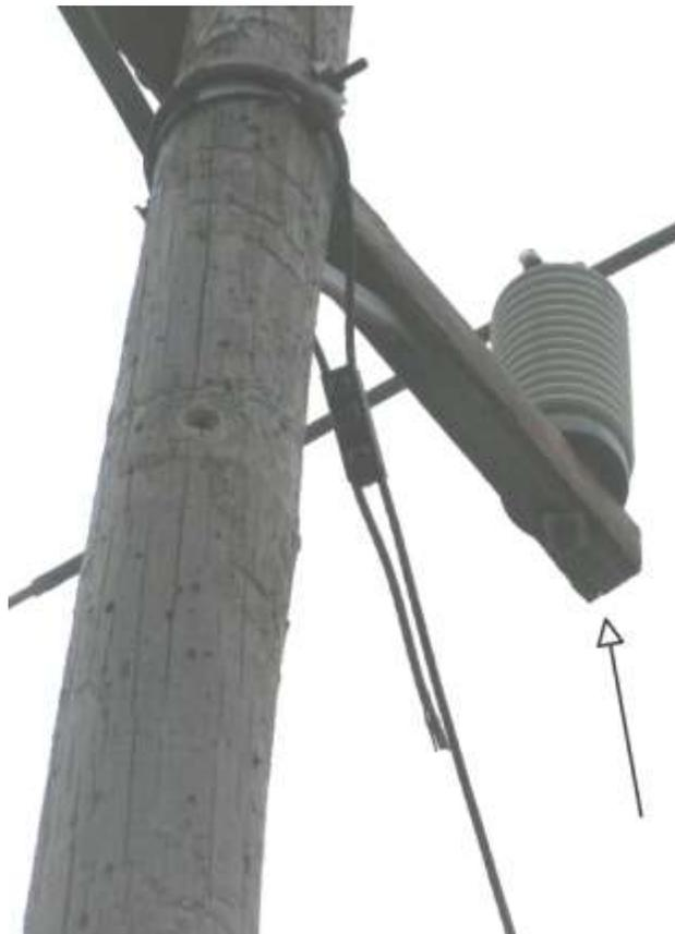
**Figure 10 – 18L - Split crossarm and nonstandard guy wire**
