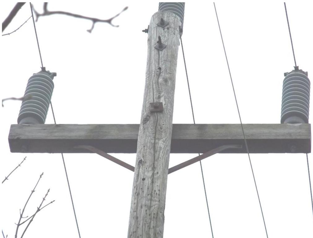
**Figure 5 – 12L - Pole showing checking around bolts**
