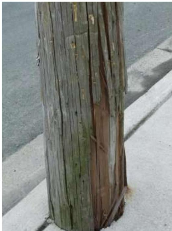
**Figure 2 – 12L - Pole showing shell separation and damage**
