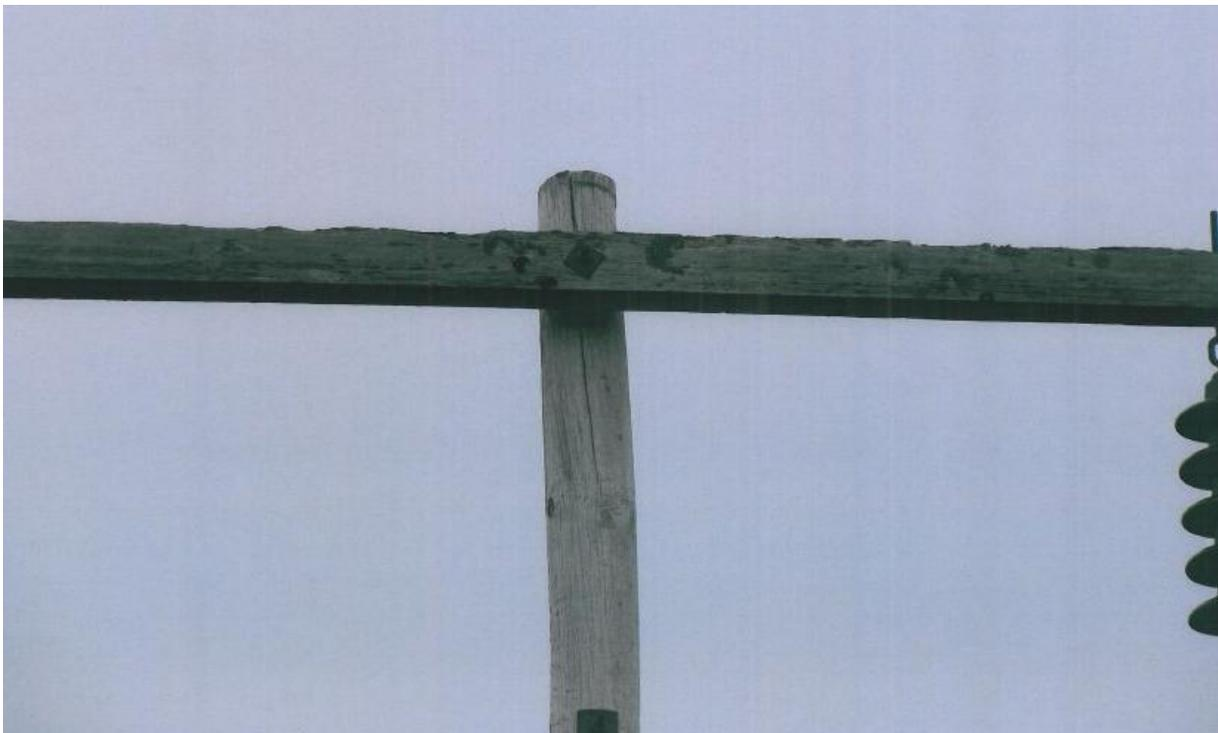
**Figure 12 – Deteriorated pole and crossarm 21L**
