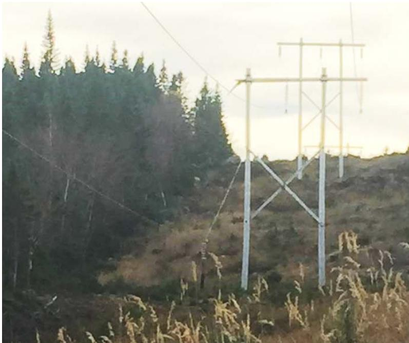
**Figure 4: 2017 Outage Conductor Falls to Ground**
