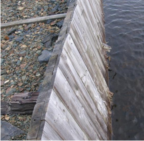
Figure 6 - Misaligned Timber Facing with Ice Damage
