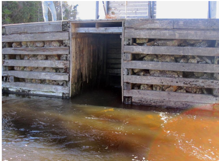
Figure 3 - Long Pond Dam (Deteriorated Outlet and Cribbing)
