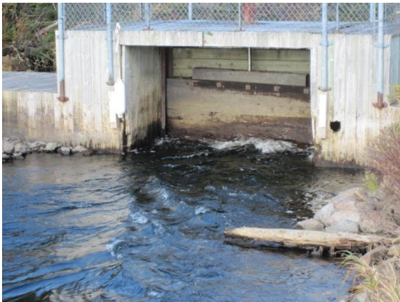
Figure 7 – Deteriorated Wood and Misaligned Gate
