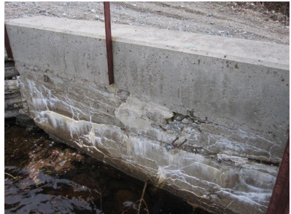
Figure 4 – Deteriorated Concrete on Upstream Face
