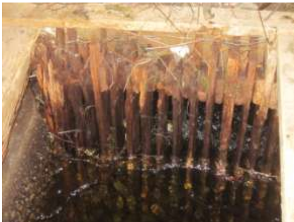
Figure 1 – Deteriorated Trash Rack
