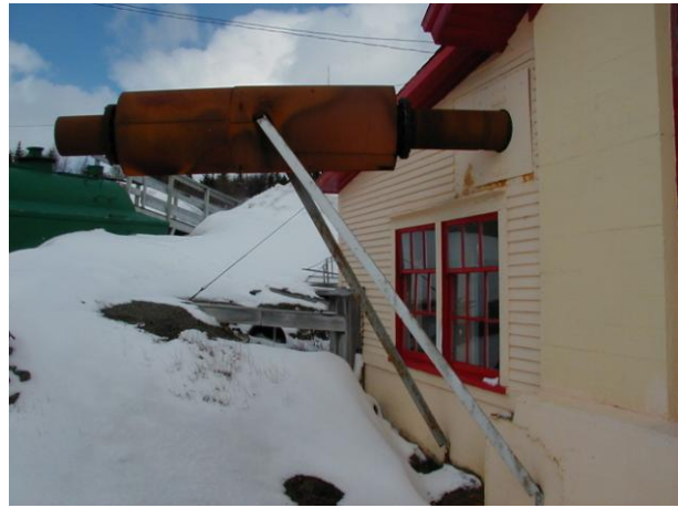
Corroded Exhaust Muffler
