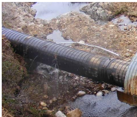
Figure 1 - Undermined Penstock
