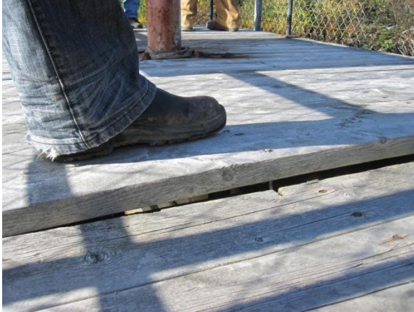
Figure 5 – Results of Settling Foundation
