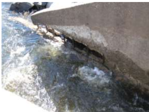
Figure 10 – Deteriorated Wingwall Concrete
