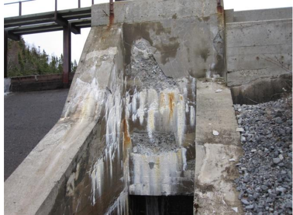
Figure 2 – Deteriorated Concrete on Sluice
