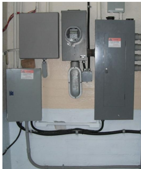
Figure 4 – AC Panels & Meter
