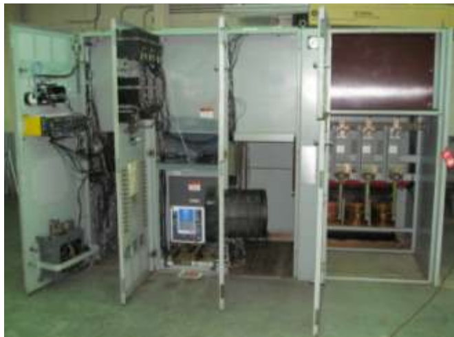
Figure 6 – Switchgear with Doors Open
