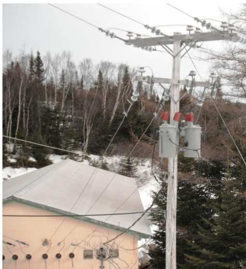
Figure 3 – Station Service Transformers
