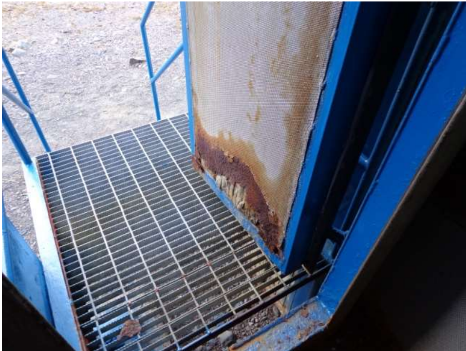
Figure 2 – Corrosion Damage Intake Plenum Door
