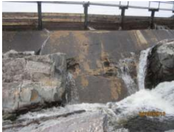
Figure 8 – Concrete Deterioration
