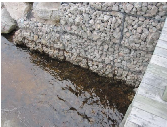
Figure 14 – Corroded Gabions - Downstream
