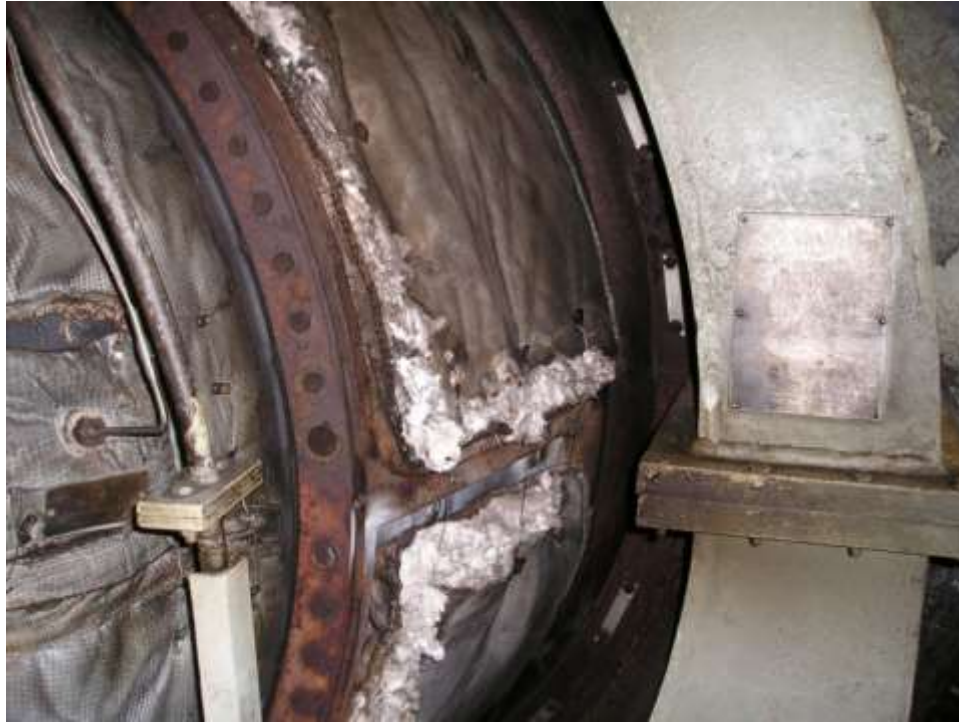
Figure 3 – Insulating Blanket Damage
