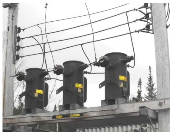
Figure 4 - Station Service Transformers
