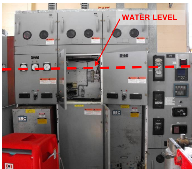
Figure 2 - Damaged Switchgear
