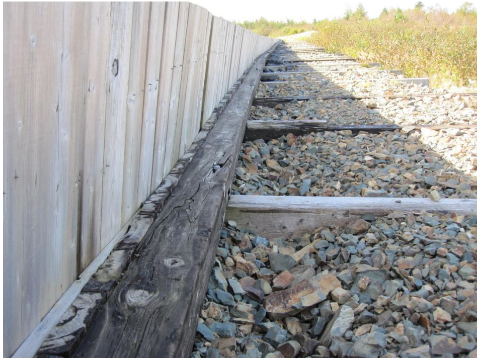
Figure 8 - Deteriorated Timbers with Erosion of Rockfill from Overtopping
