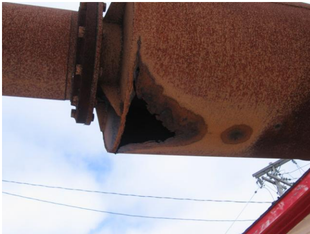
Hole In Muffler
