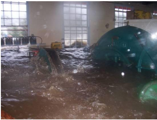
Figure 1 - 2m of water in the powerhouse (Note: Turbine still spinning)
