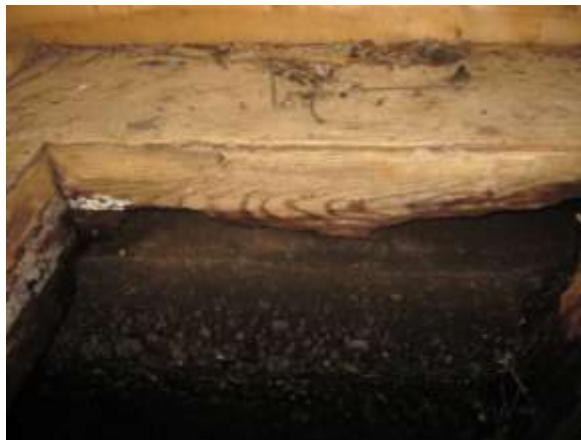
Figure 2 – Deteriorated Timber Deck
