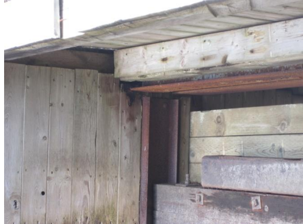
Figure 6 – Misalignment Due to Settling
