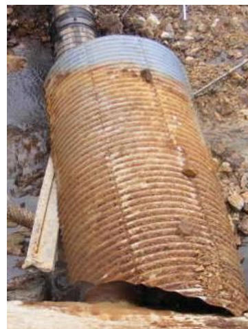
Figure 2 - Damaged multi-plate culvert (Rust indicates extent of the rockfill)
