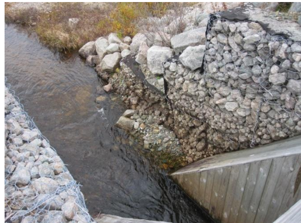
Figure 13 – Corroded Gabions - Upstream
