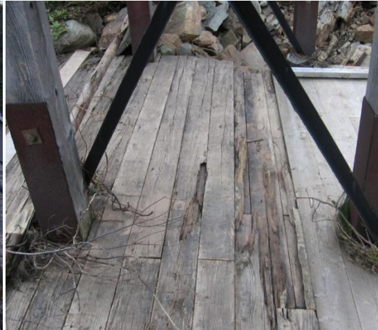
Figure 2 - Long Pond Dam (Deteriorated Decking)
