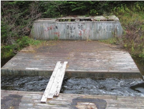
Figure 9 – Evidence of Fires and Crossing Using Structure Timbers
