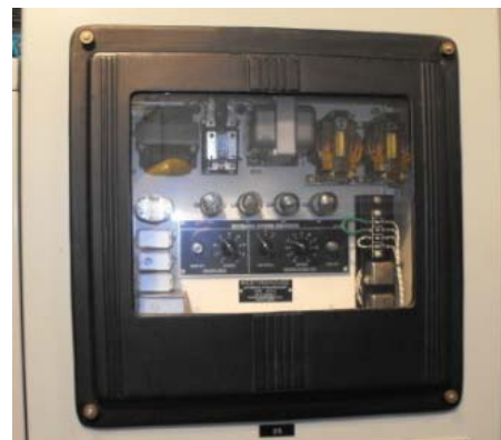
Figure 6 - XT7 Auto-synchronizer
