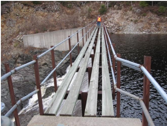
Figure 3 – Missing and Substandard Railing
