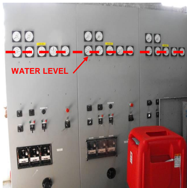
Figure 3 - Damaged Protection and Control
