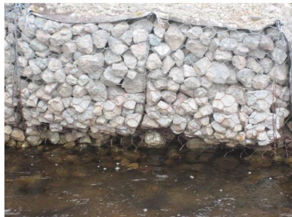
Figure 15 – Corroded Gabions - Downstream
