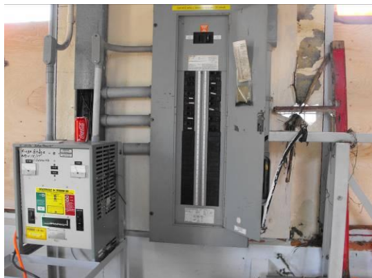
Figure 4 - DC Distribution Panel and Battery Charger
