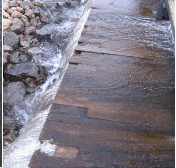
Figure 7 - Delaminating Spillway Decking
