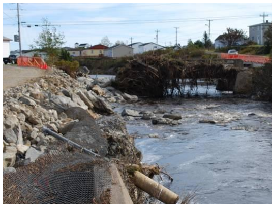
Figure 6 - Erosion, Plant Access Road (Downstream of Plant)
