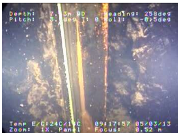
Figure 15 – Gate Guide (Note: Deteriorated Concrete behind gate guide)
