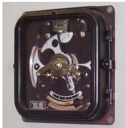
Figure 1 - BB Voltage Regulator
