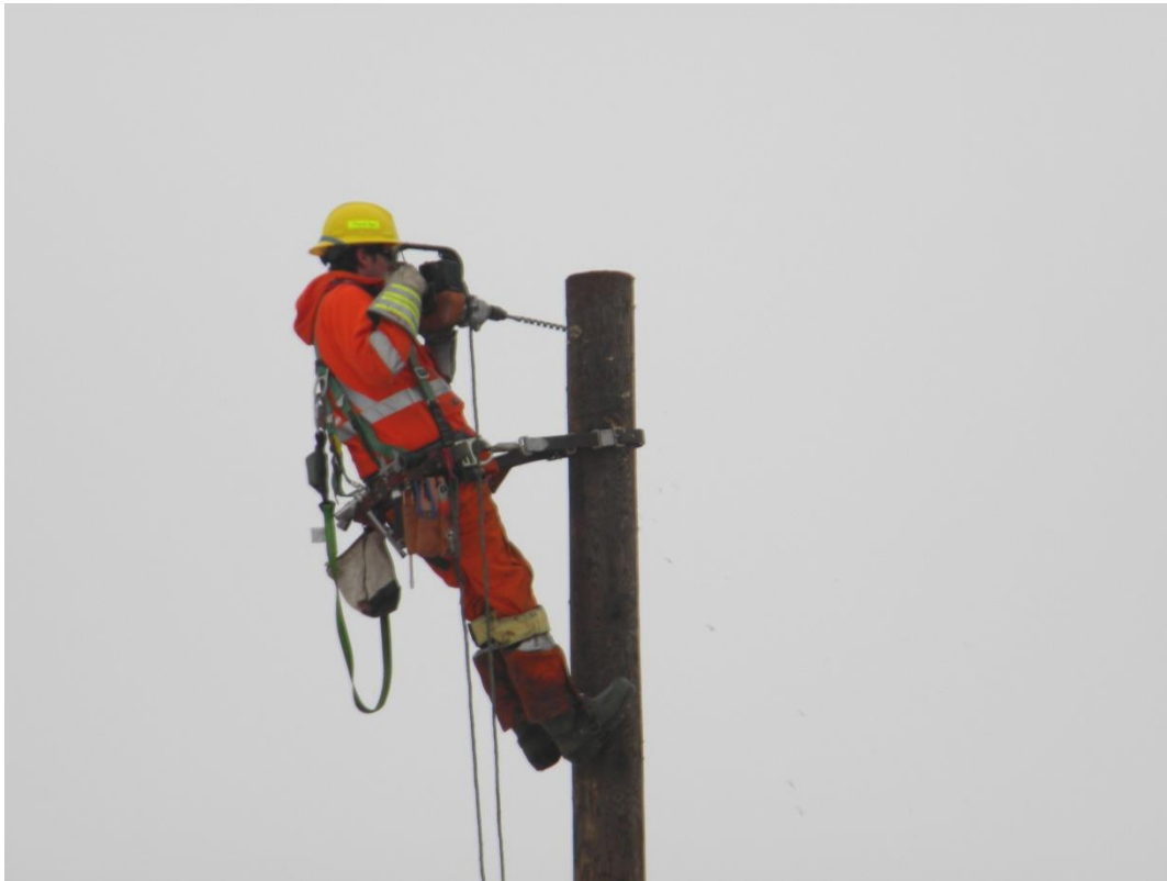
Preparing Pole to Attach Fittings
