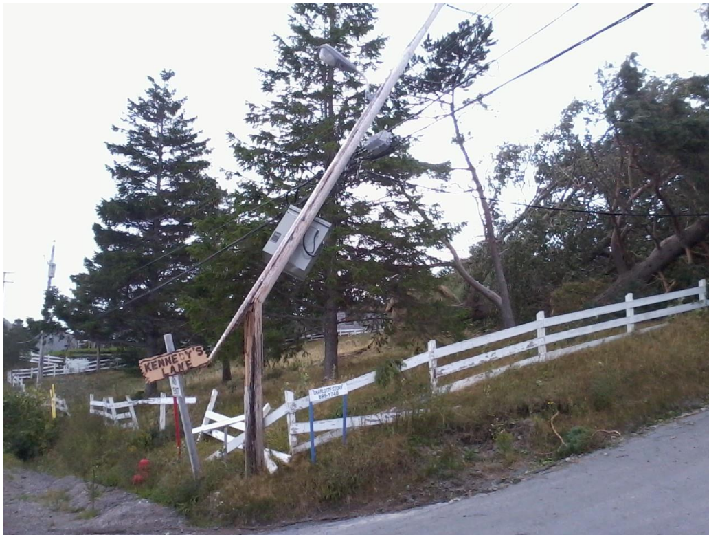
Pole Cracked, Kennedy's Lane, Holyrood
