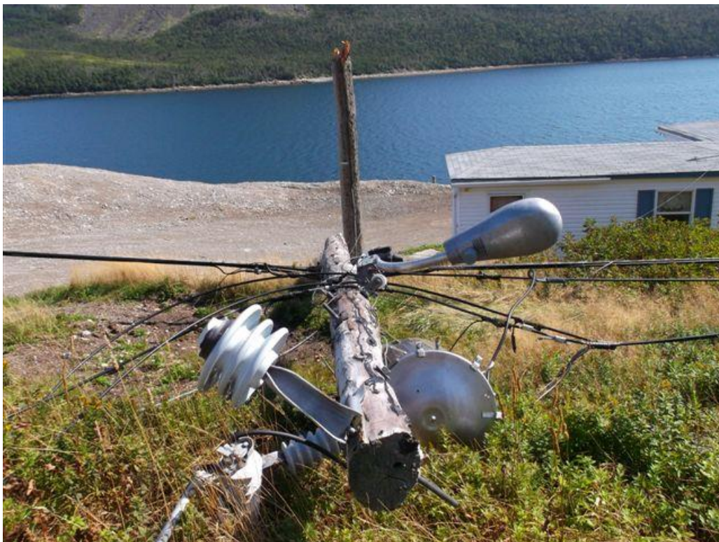
Broken Pole, Ship Cove
