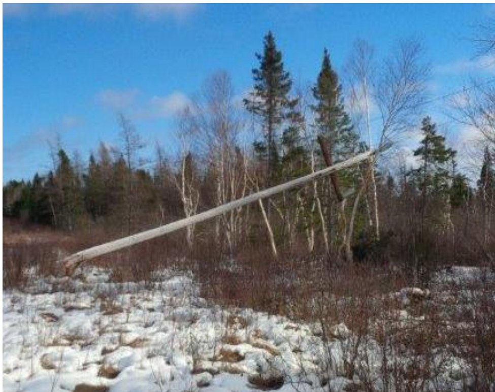
105L Transmission Structure Broken at Base of Pole
