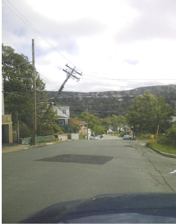
Main Line Pole Leaning into Street, St. John's
