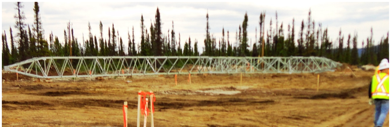
Photo 8.1: Transmission Tower Erection and Foundations. Assembled single HVac tower unit. (July 17, 2014)
