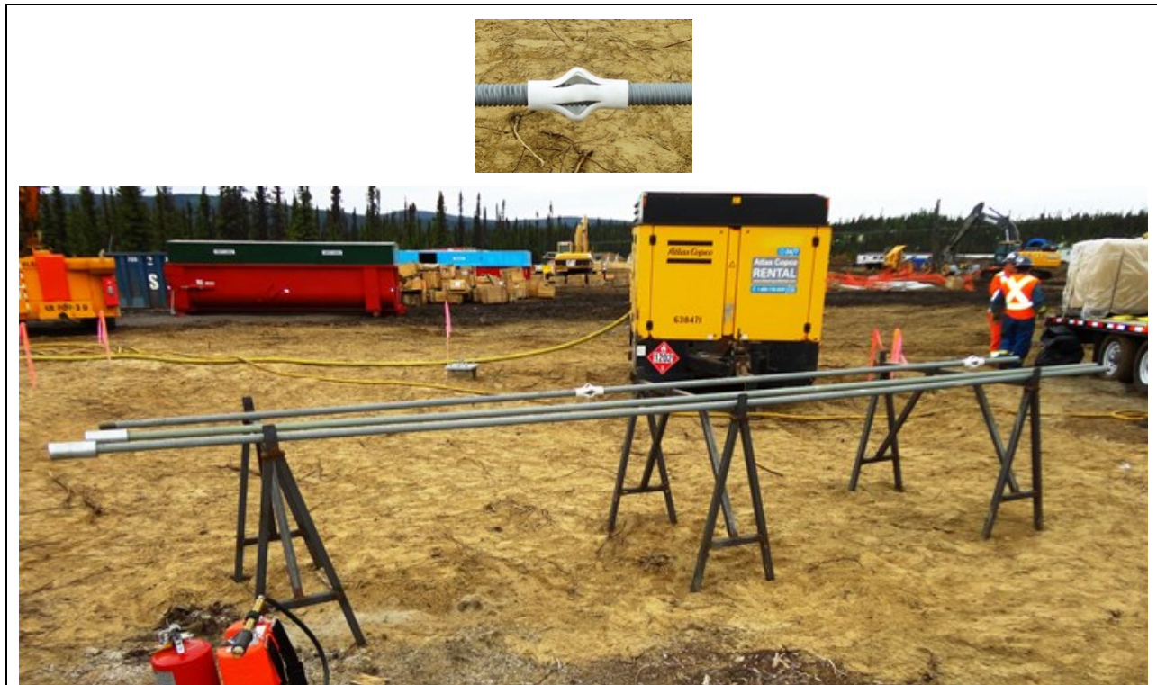
Photo 8.5: Transmission Tower Erection and Foundations. Ground anchorage assembly, complete with couplers. Inset shows a typical plastic centralizer (July 16, 2014)
