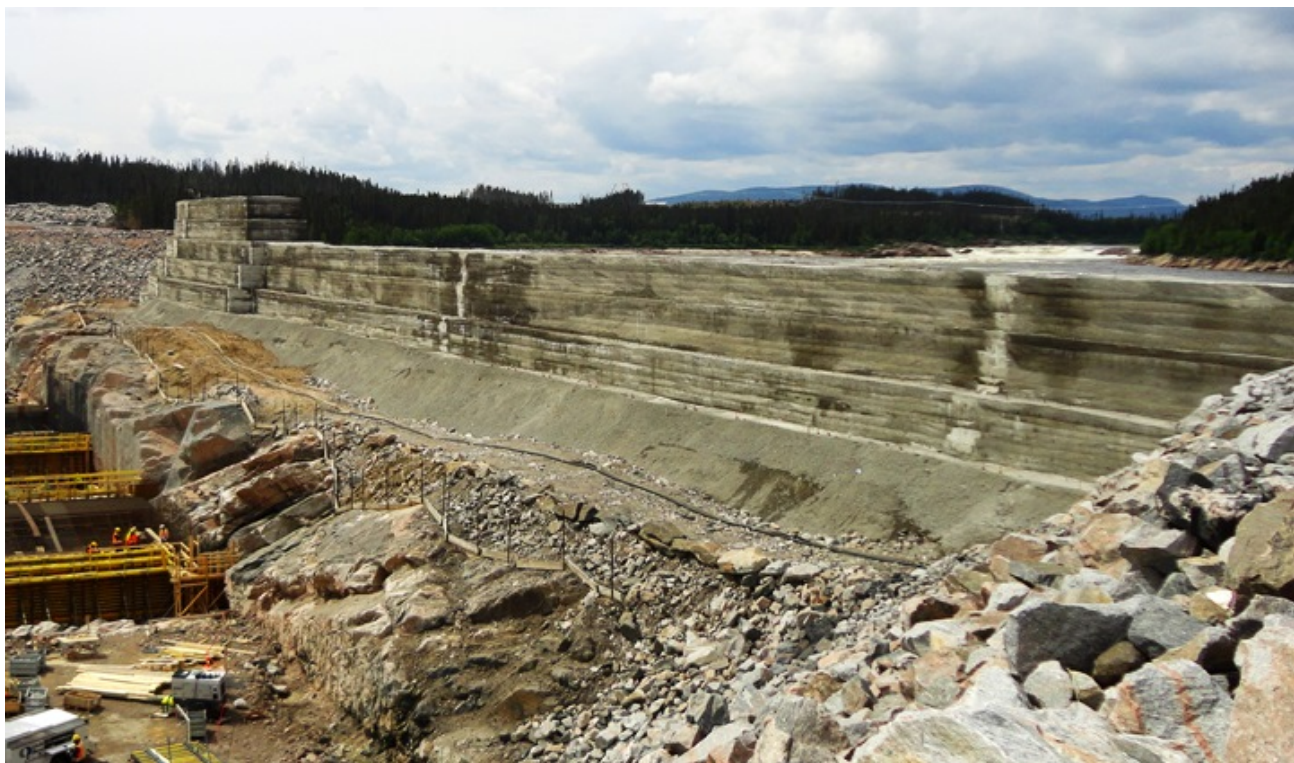
Photo 6.3: RCC cofferdam above the spillway left wall. Note the localized blasting overbreak of the spillway rock slope caused by block sliding along pervasive foliation planes. (July 17, 2014)
