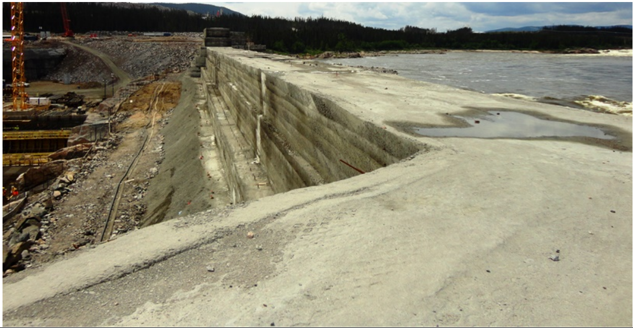
Photo 6.4: RCC cofferdam above spillway left wall. (July 17, 2014)
