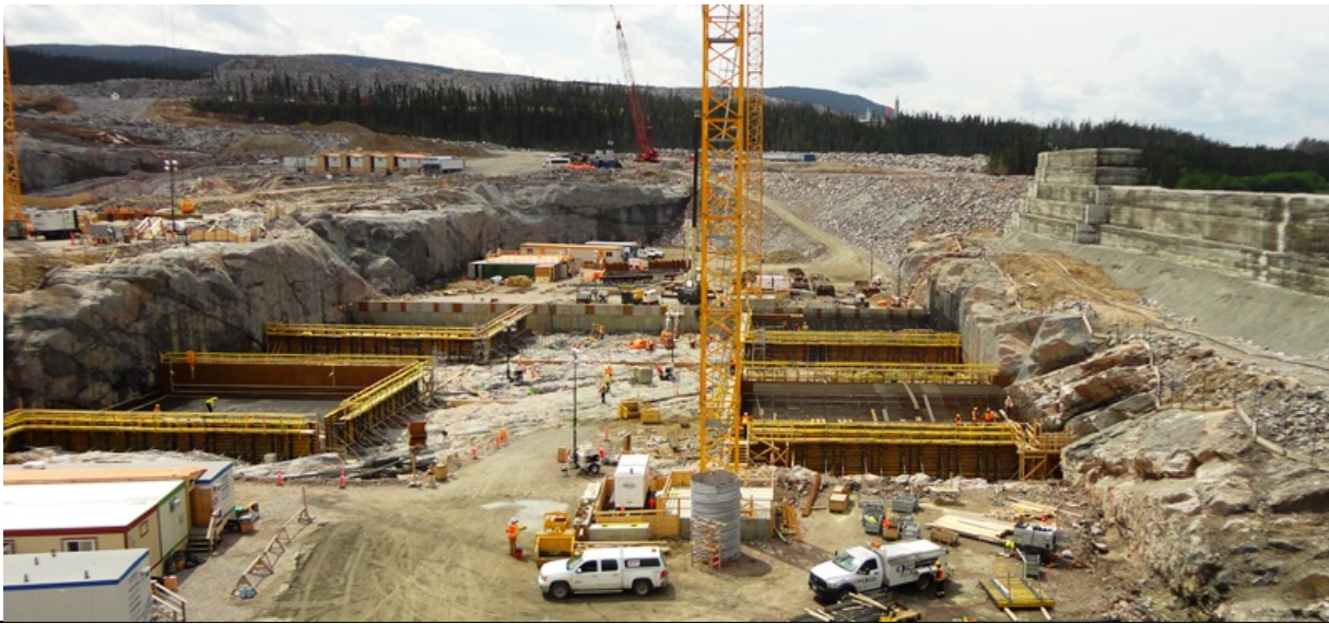
Photo 6.2: Spillway base slab. Formwork for first four blocks of the base slab. (July 17, 2014)
