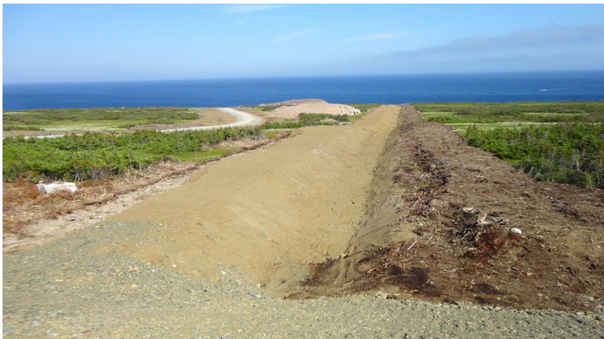
Photo 2.7: Forteau Directional Drilling. Excavated trench for the three cables between the transition compound and the drilling site. (July 15, 2014)
