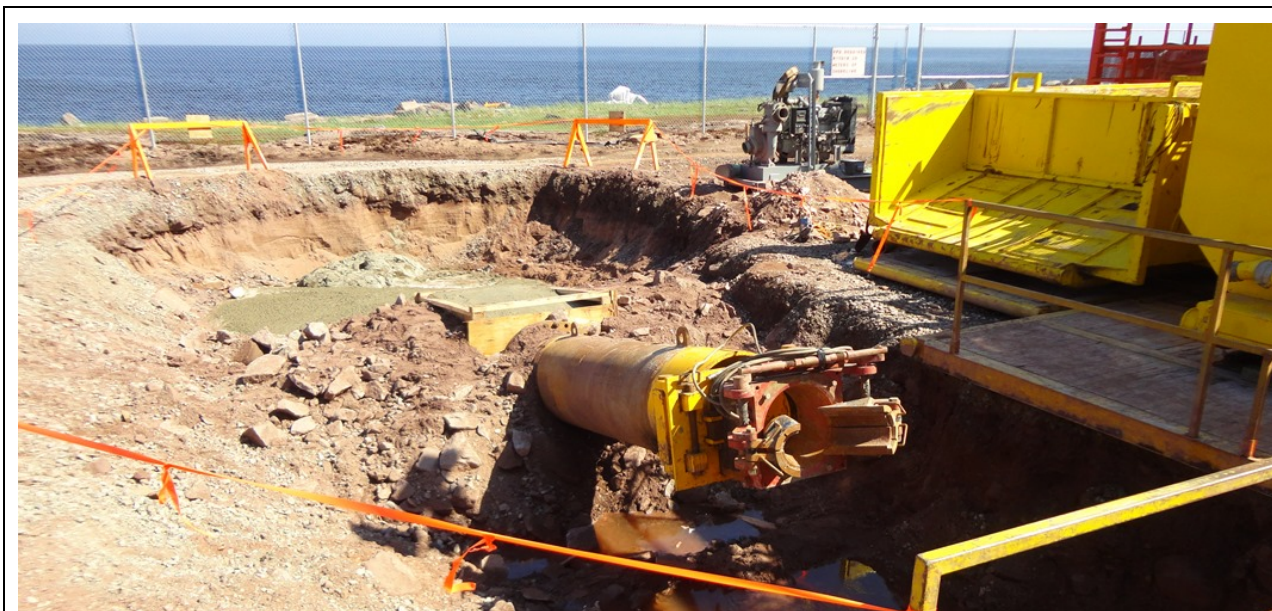
Photo 2.3: Forteau Directional Drilling. , Photo of borehole Forteau 2 showing the 30 inch casing collar. (July 15, 2014)
