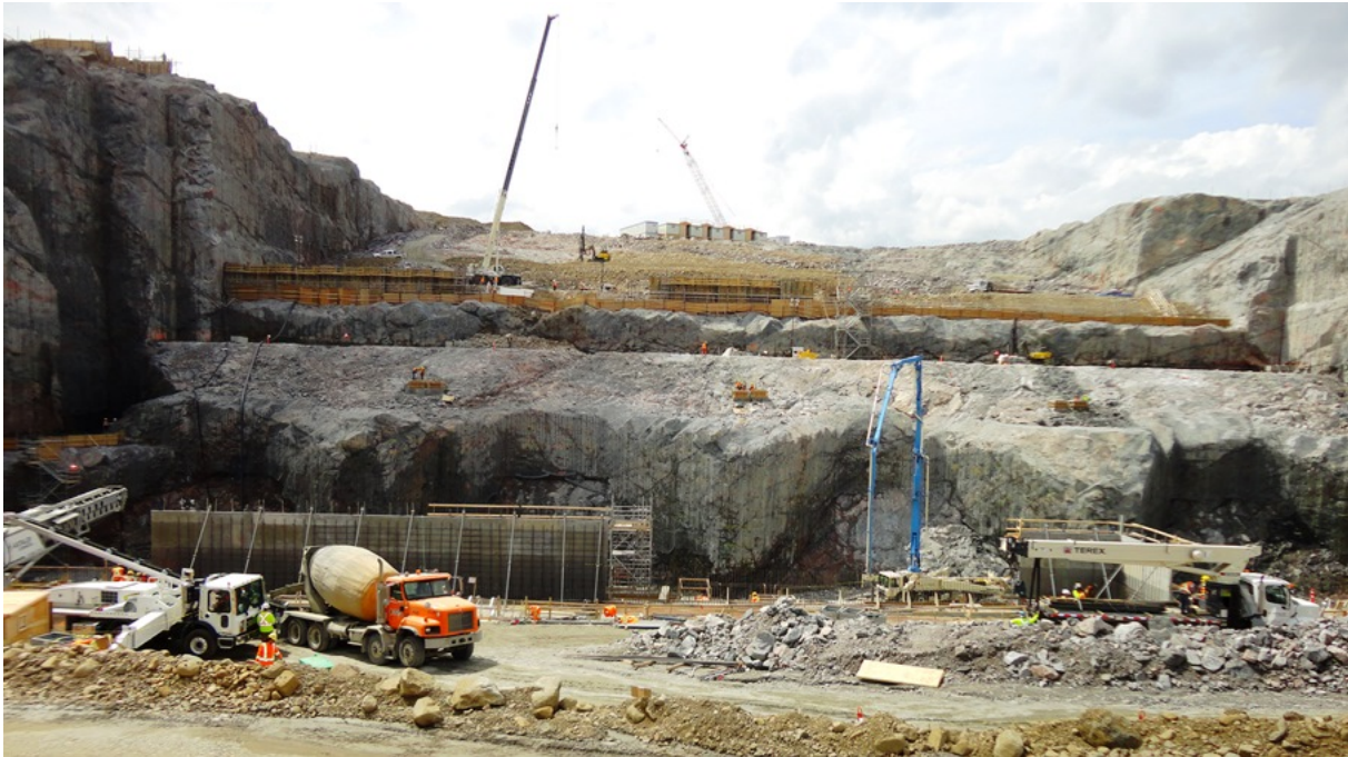
Photo 6.6: Powerhouse excavation, view looking upstream. The excellent control blasting results are visible in the rock noses between the unit cut-outs. (July 16, 2014)
