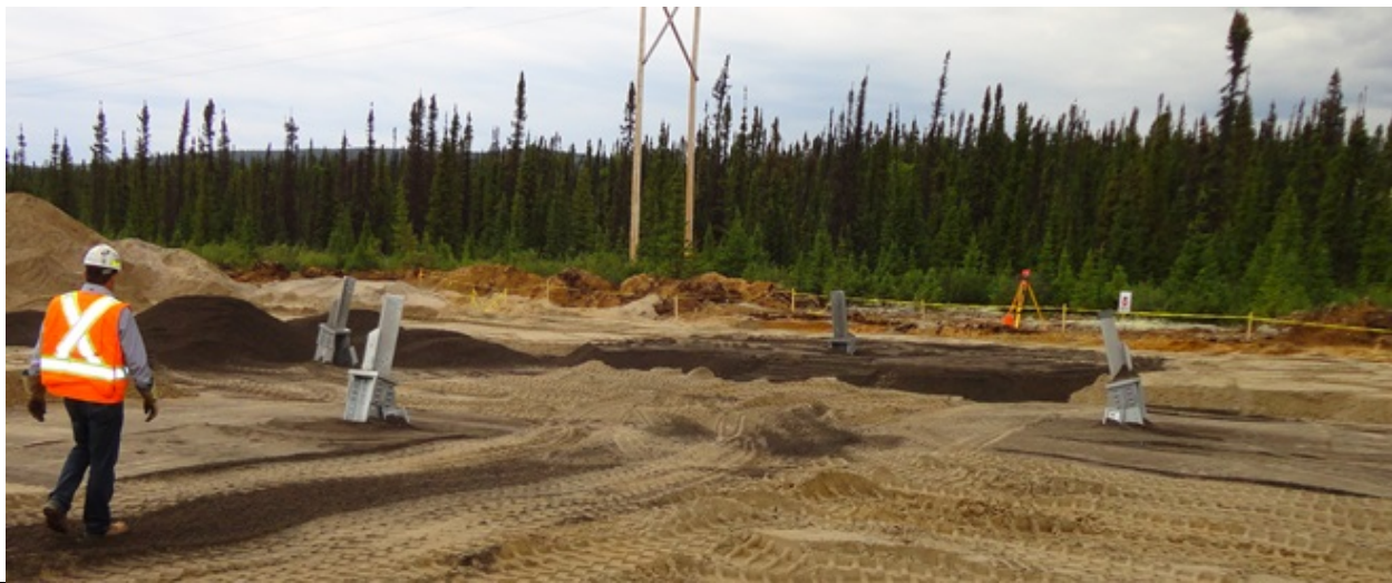
Photo 8.4: Transmission Tower Erection and Foundations. Tower footings installed and backfilled (four legged tower) (July 16, 2014)
