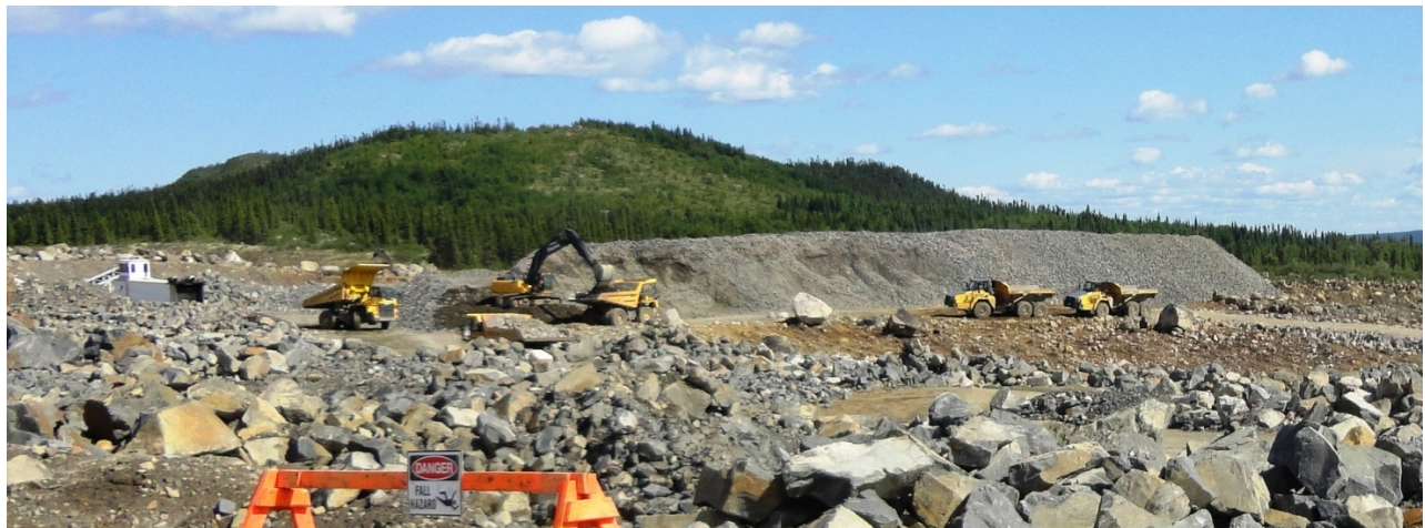
Photo 10.1: Churchill Falls New 315 kV substation and switchyard. Loading processed fill. Note stockpile of processed fill in the background and blasted rock in foreground. (July 18, 2014)
