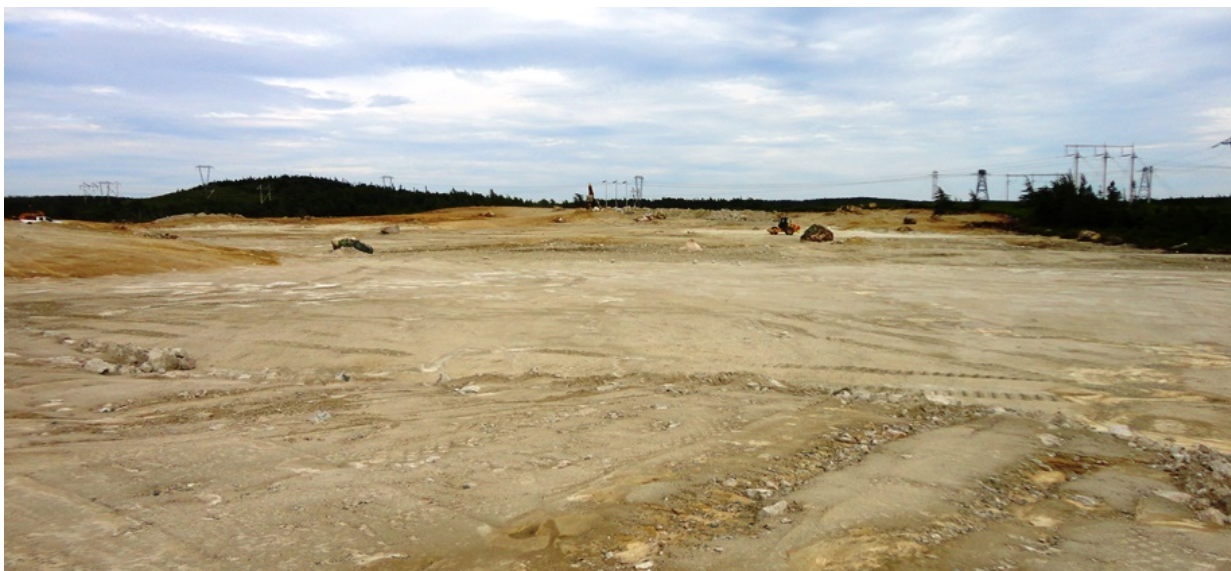
Photo 1.2: Soldier's Pond site; placing compacted fill to grade at east half of the site. (July 14, 2014)
