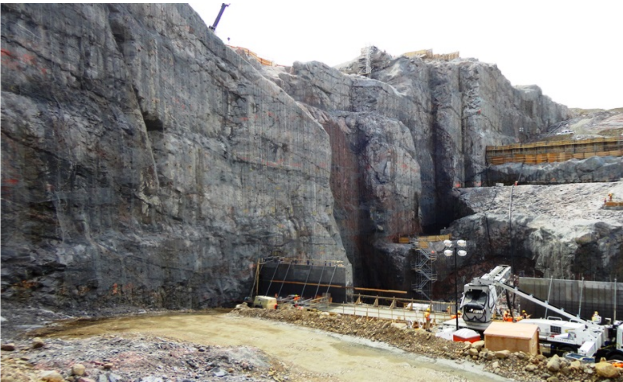
Photo 6.5: Right rock slope at powerhouse. Note the excellent quality of the line drilled excavated rock walls. A single fallout of a small wedges has caused a very localized overbreak feature. (July 17, 2014)
