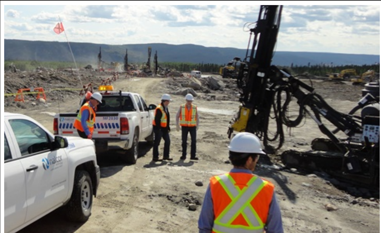
Photo 10.2: Churchill Falls New 315 kV substation and switchyard. Blast hole drilling in bedrock. (July 18, 2014)
