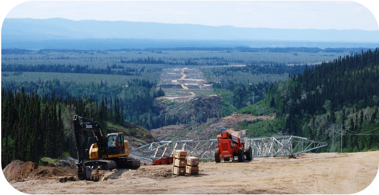
Work on the HVac steel towers which will be installed on the transmission line between Muskrat Falls and Churchill Falls (Labrador Transmission Assets).
