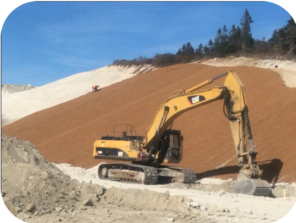
Installation of erosion control blanket (coconut blanket)
