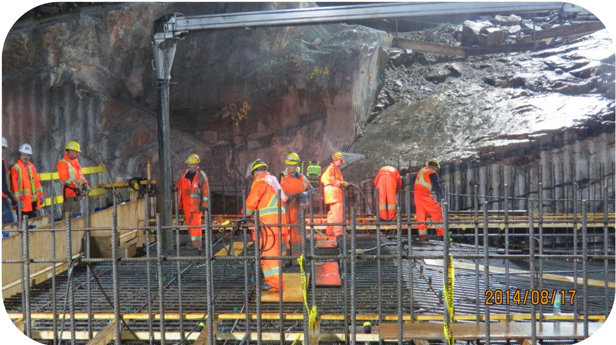
Concrete placement commenced on August 17, 2014, at the Muskrat Falls spillway structure. The powerhouse/intake and spillway structures combined will require 560,000 cubic metres of concrete.
