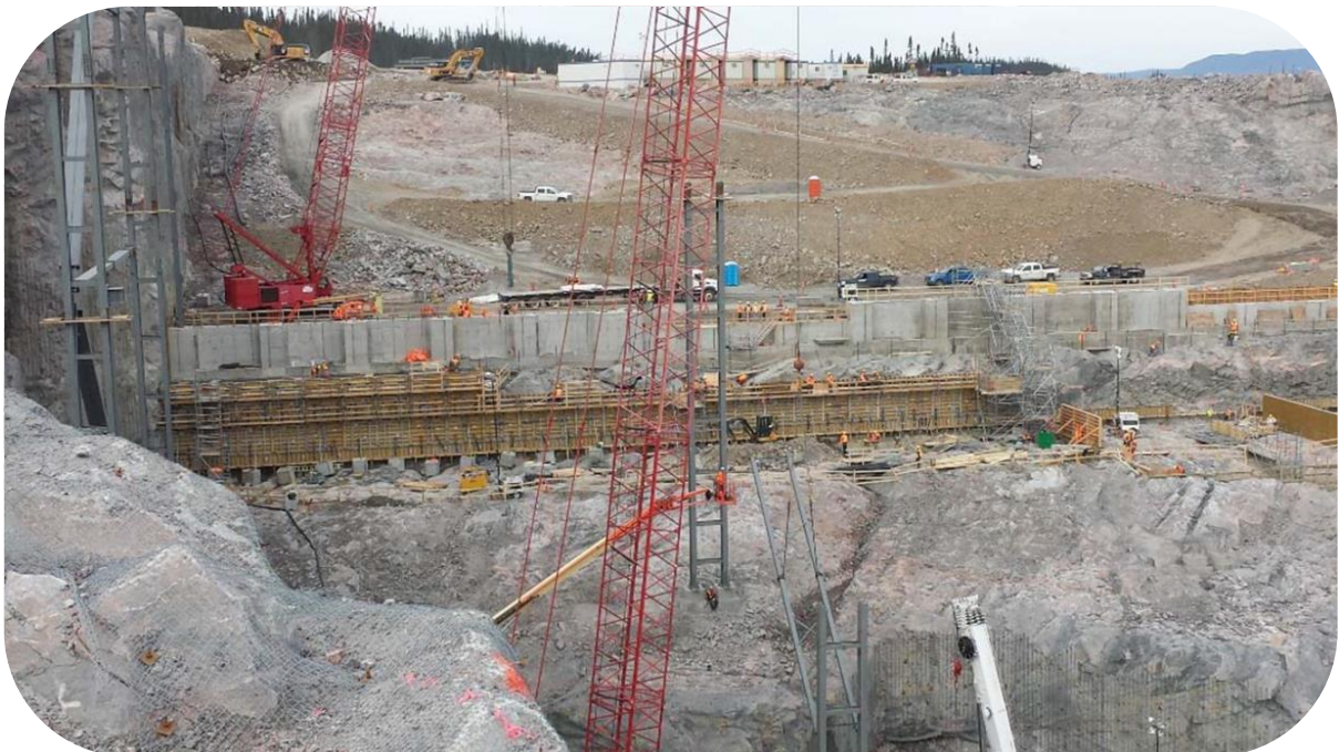
Assembly of the Integrated Cover System (ICS) for the powerhouse area.
