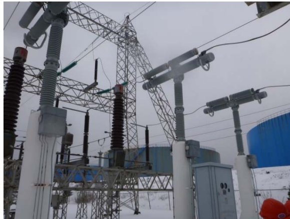
Illustration 3.4: Air-Blast Circuit Breaker B1L17
