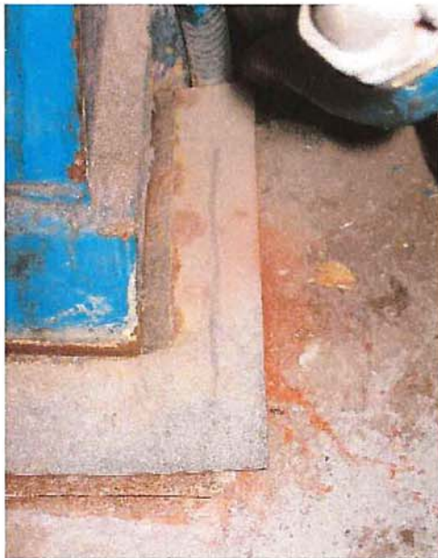
Figure 2 Generator Shim – RHS Collector End
