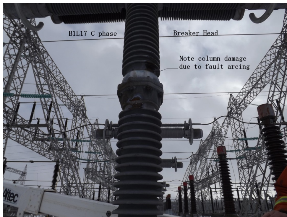
Figure 2-5d: B1L17 Vertical Column Arcing Damage
