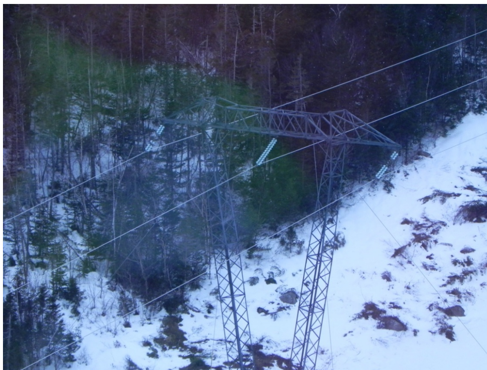
Figure 2-9a: Picture of TL217 Structure 282 with Damaged Insulators
