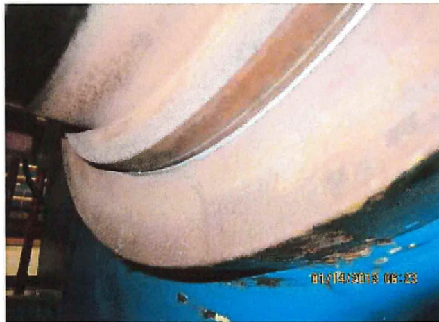
Figure 4 Bearing #4 – lower oil deflector clearance
