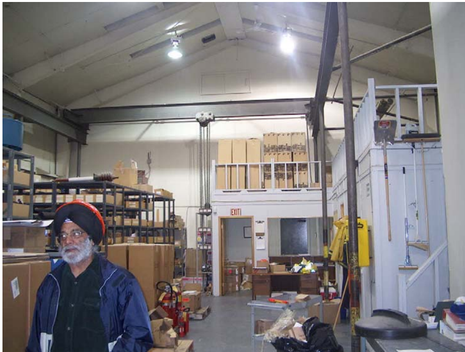
Photo 14 Interior of Warehouse showing General Clutter, Overhead Crane and Asbestos Sheeting in End Wall.
