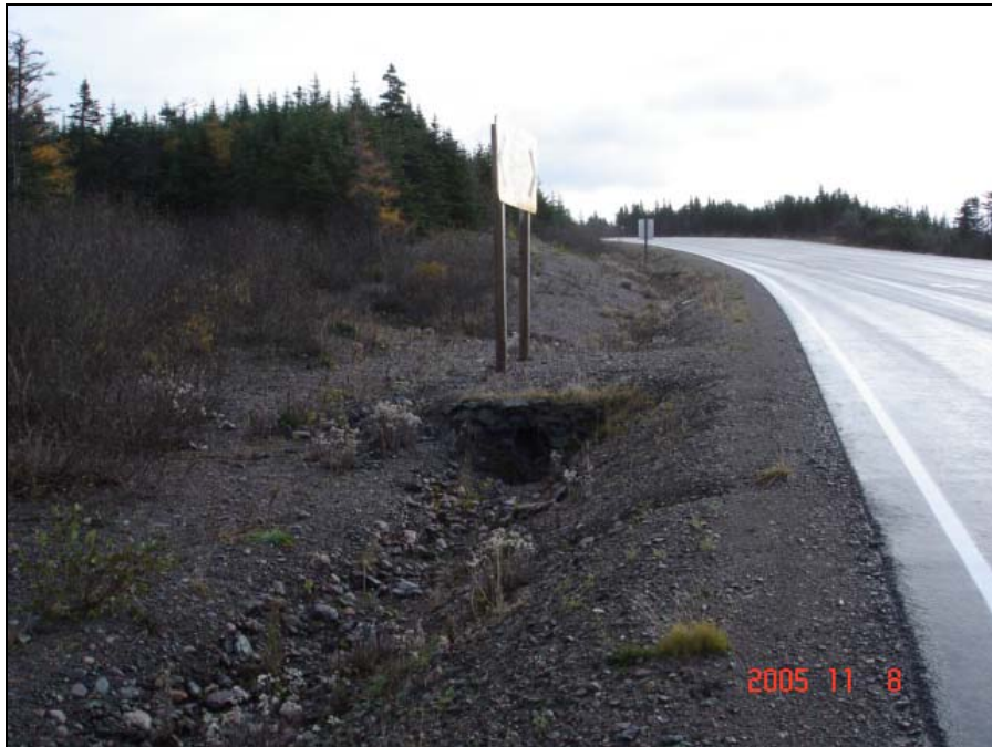
This highway location shows a very narrow shoulder (less than 0.5 m). Roadside vehicles which may be parked at this location would pose a hazard for on-coming traffic.
