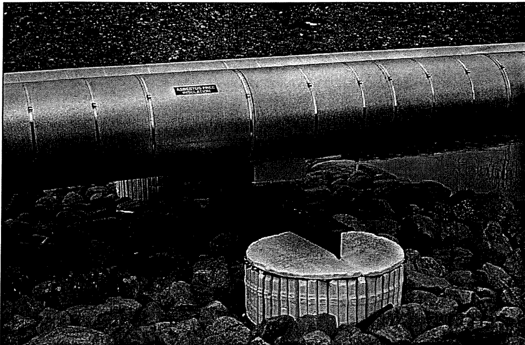
Photo 3: Main Trunk Line near Tank 3. Pipe saddle moved longitudinally and previously repaired.
