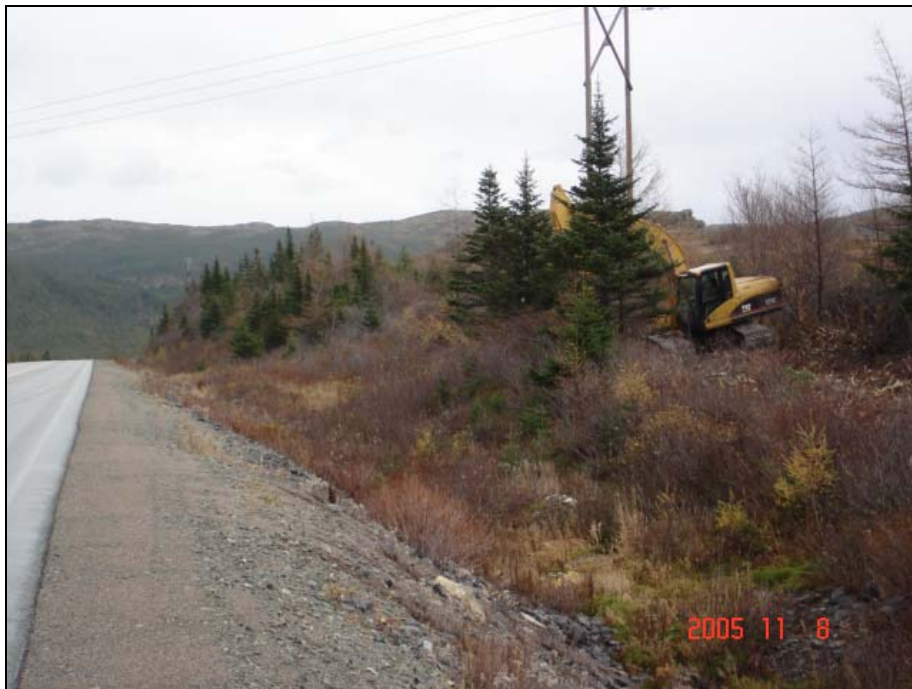
This section of the highway shows a steep-sloped roadside embankment, making offloading at this location very difficult. In this case, the excavator was offloaded at a separate location and traveled to the transmission site.
