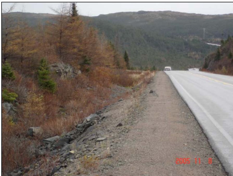
This offloading site at the crest of a hill shows a short site distance for on-coming traffic.
