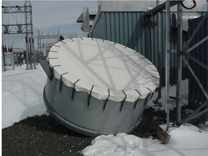
Figure 1. Microwave antenna with radome.
