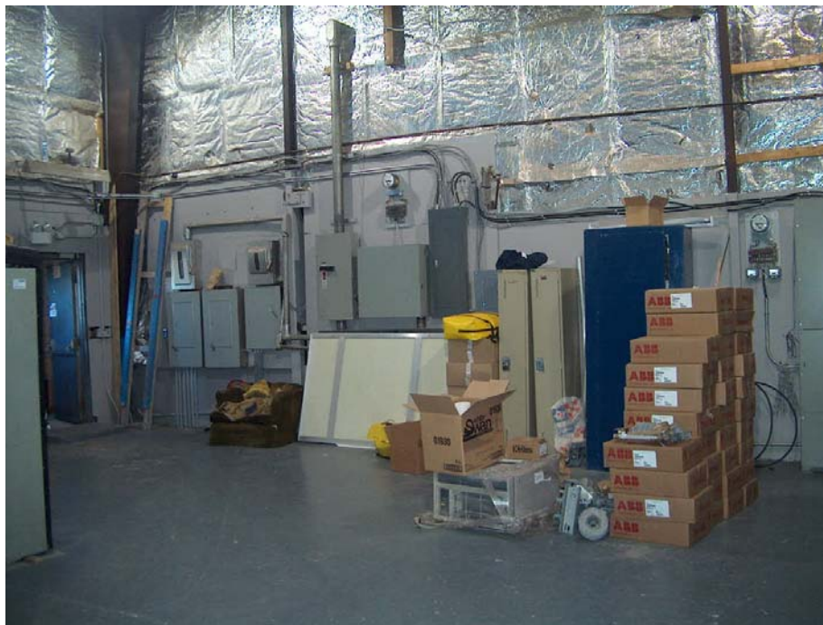
Photo 12 Interior of Line Depot Building Showing Electrical Panel Congestion
