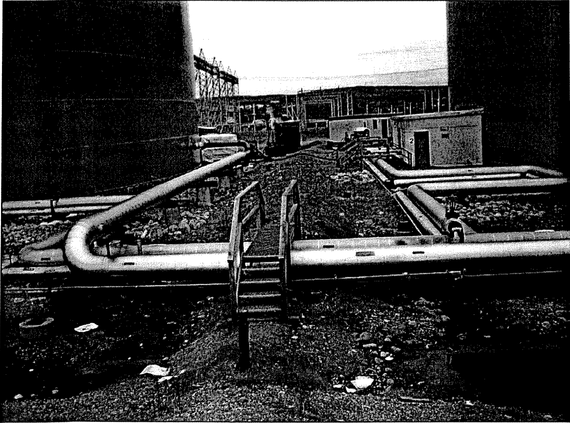
Typical installation of wooden / steel walkways.
