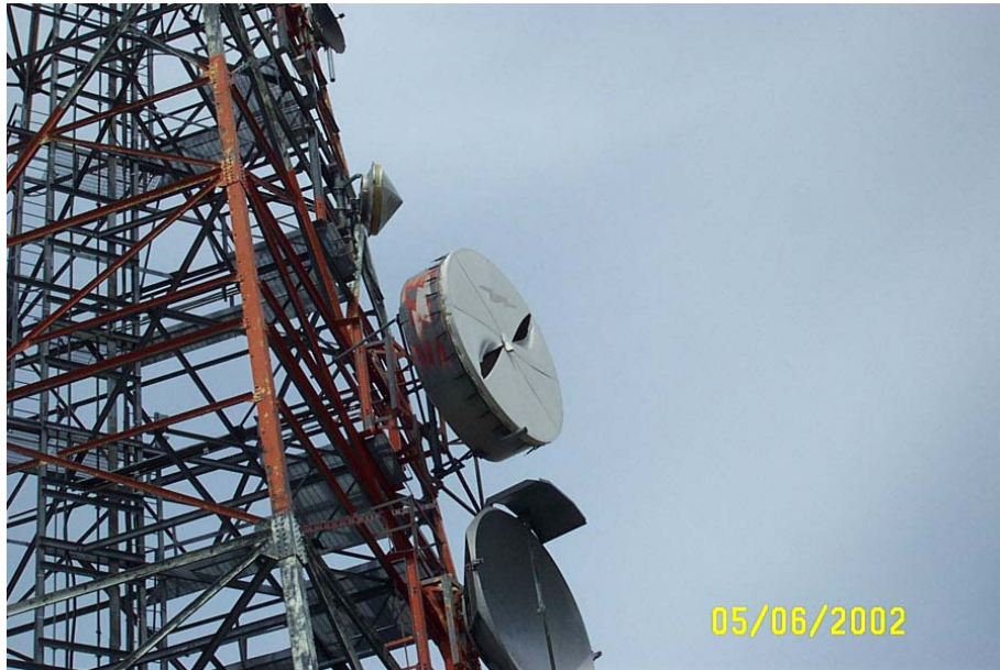
Figure 3. Heavily damaged radome.
