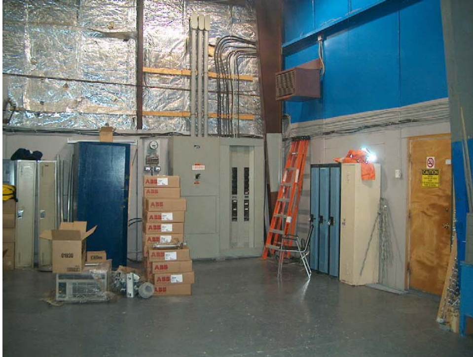
Photo 13 Interior of Line Depot Building Showing Electrical Panel Congestion on same Wall as Photo 11.
