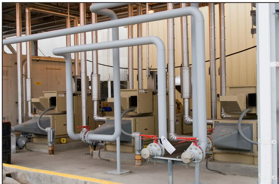
***The trona injection system features a relatively low injection rate and minimal operation and maintenance requirements.***
