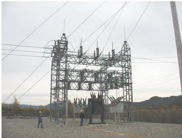
66kV Steel Structures & Bus
