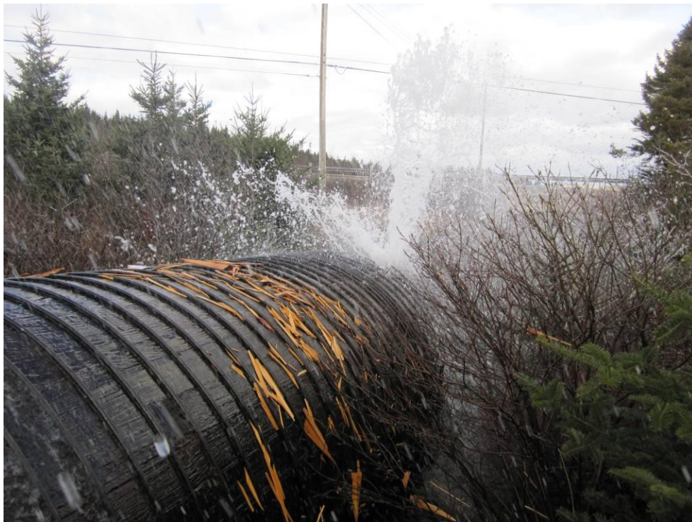
Figure 4: Major Leak (Partially repaired)
