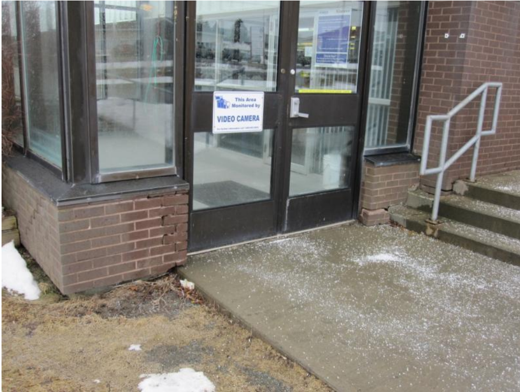
Figure 3 – Cracked Exterior Brick on Atrium
