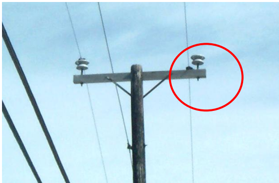
Figure 6: Broken Insulator In Service
