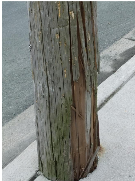
Figure 6 – 12L – Pole showing shell separation and damage
