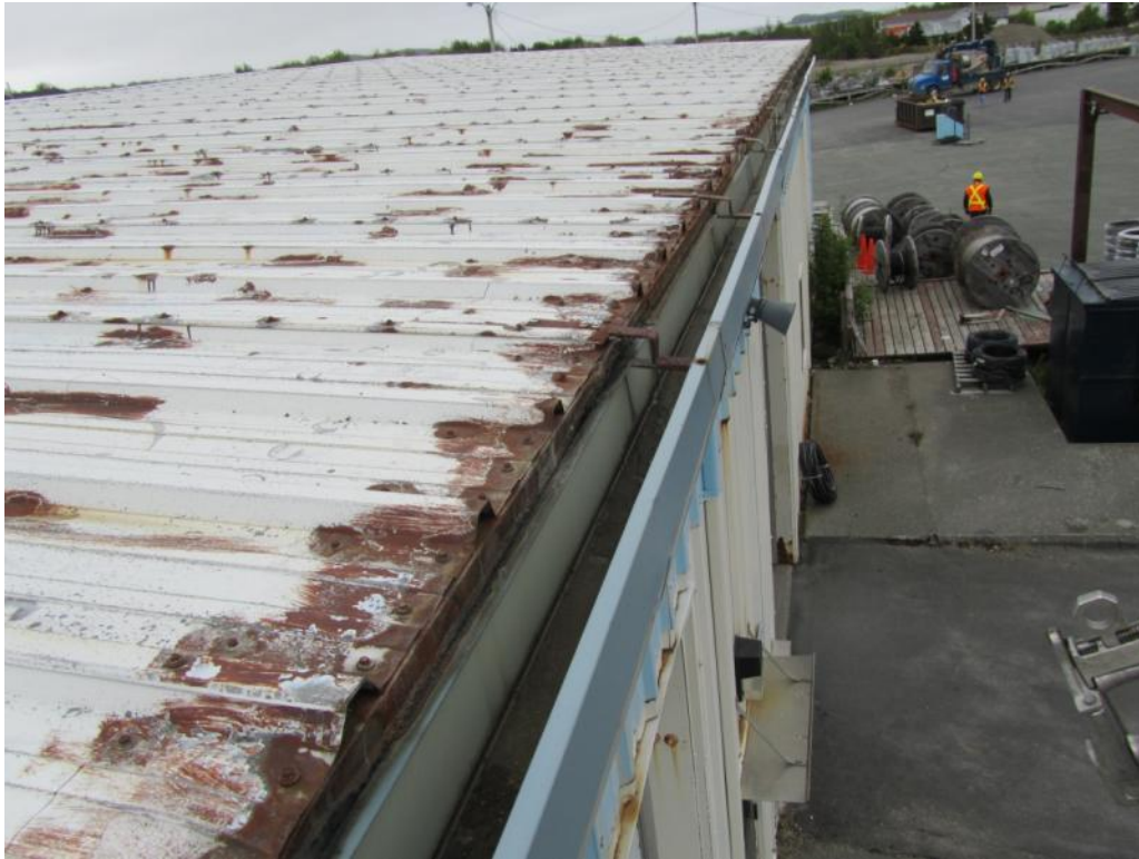
Figure 5 – Corrosion on Warehouse Metal Roof
