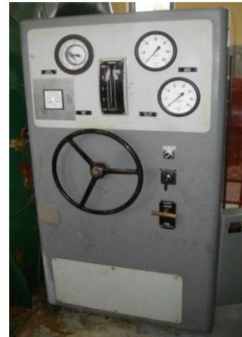
Figure 1 - Gate Positioner
