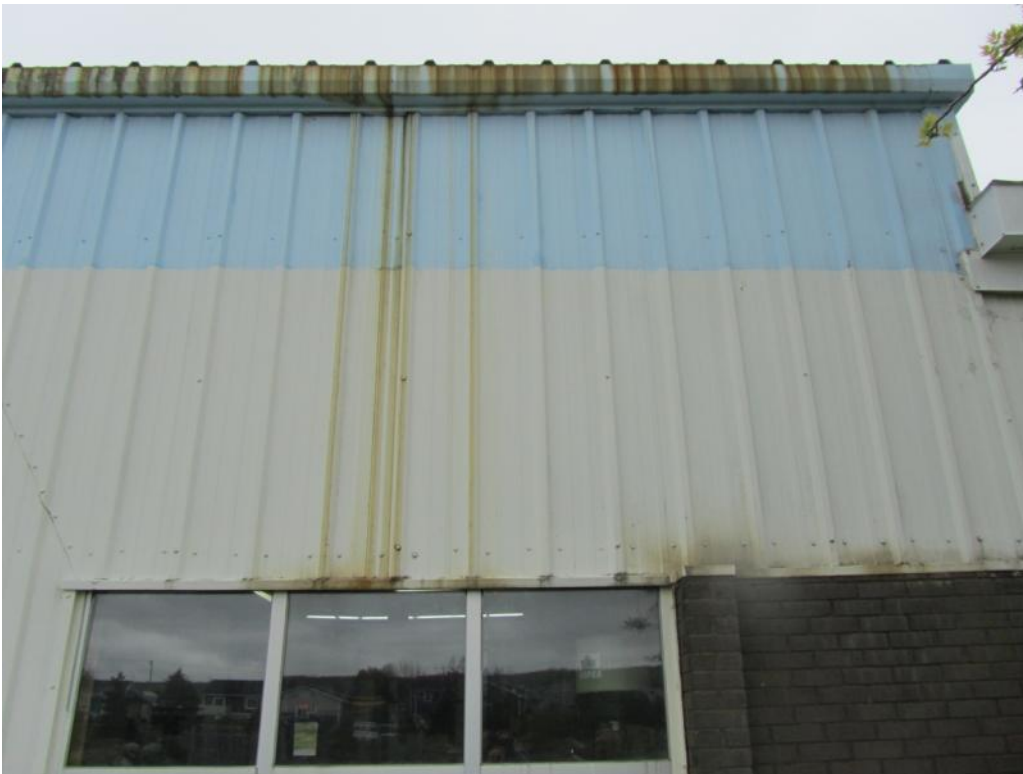
Figure 6 – Corrosion on Exterior Siding and Eave
