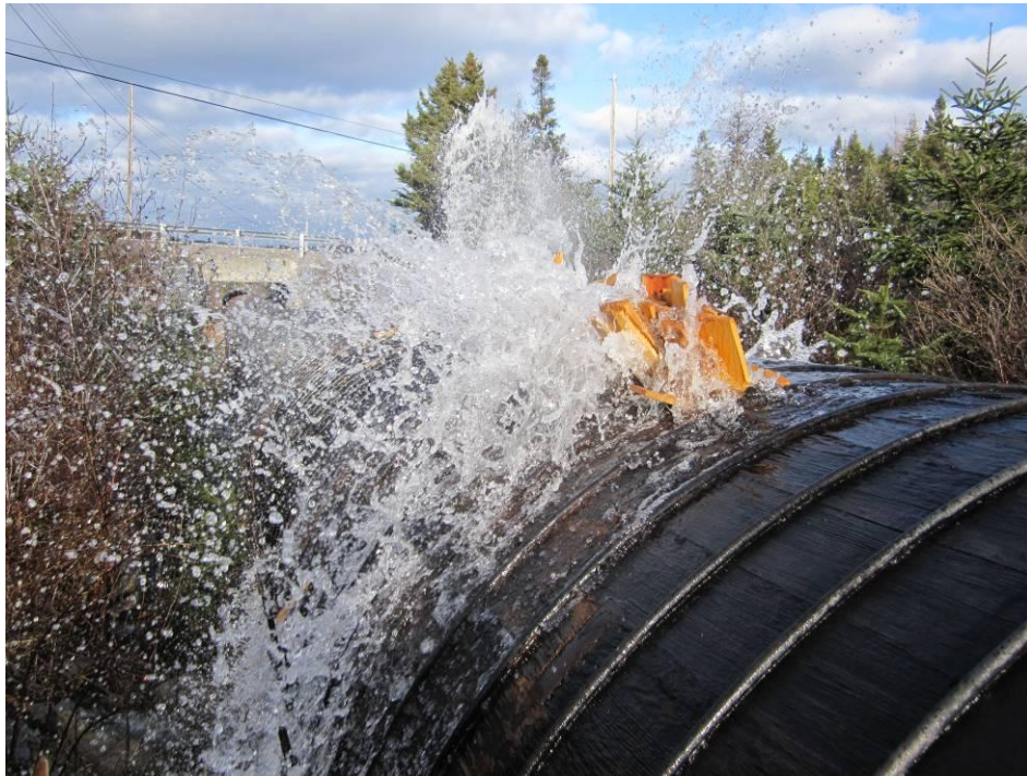
Figure 5: Blown Out Stave
