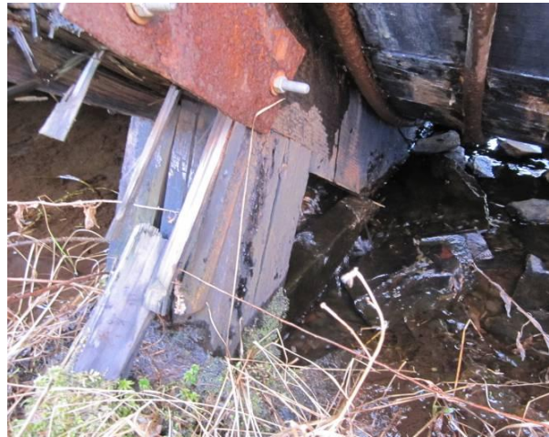
Figure 2 - Cracked Cradle
