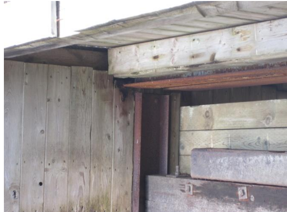
Figure 6 – Misalignment Due to Settling
