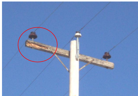
Figure 2: Rotten Crossarm
