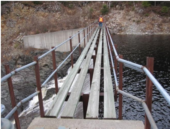
Figure 3 – Missing and Substandard Railing
