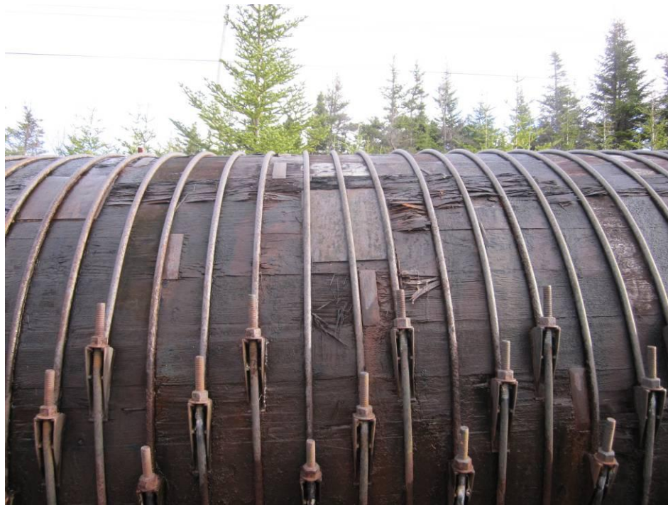
Figure 6: Repaired and Deteriorated Staves
