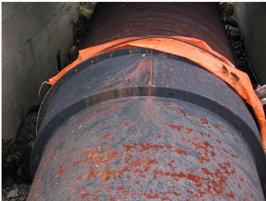
Figure 14: Woodstave/Steel Interface (Note: Deteriorated Coating)
