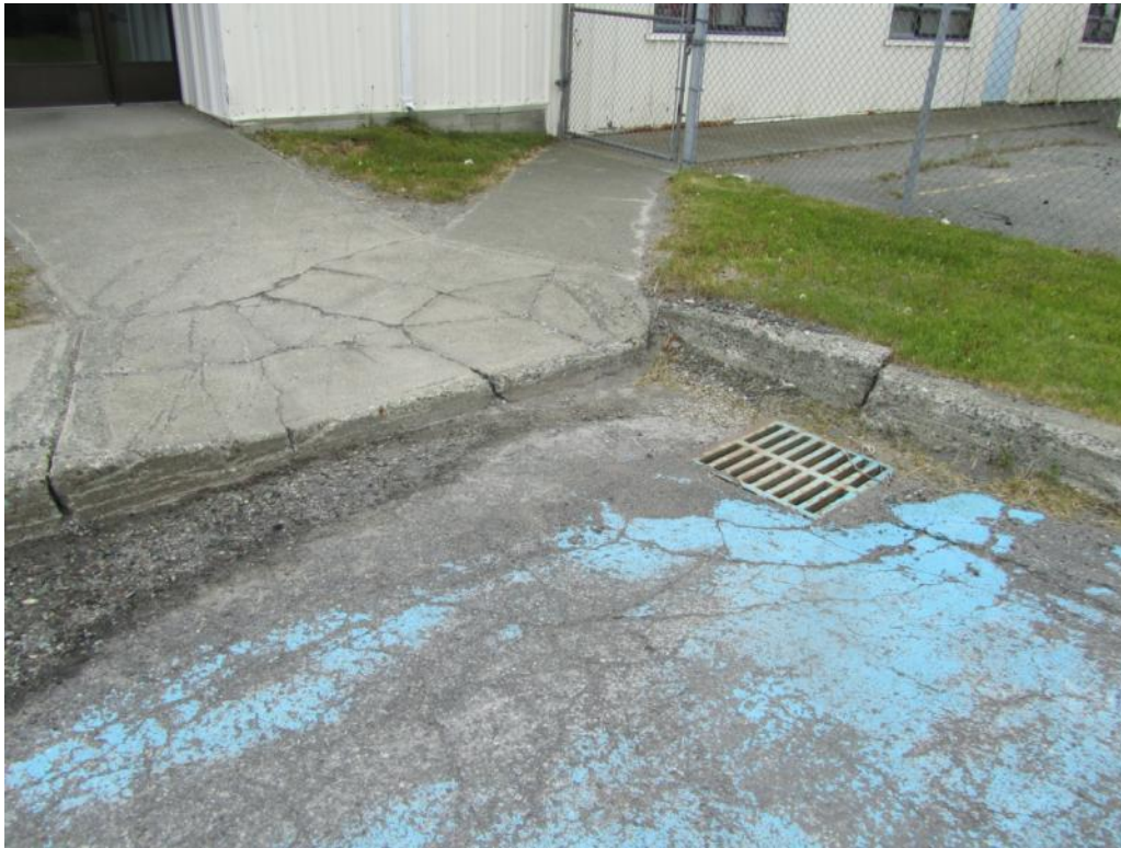
Figure 9 – Deteriorated Asphalt and Concrete Walkway
