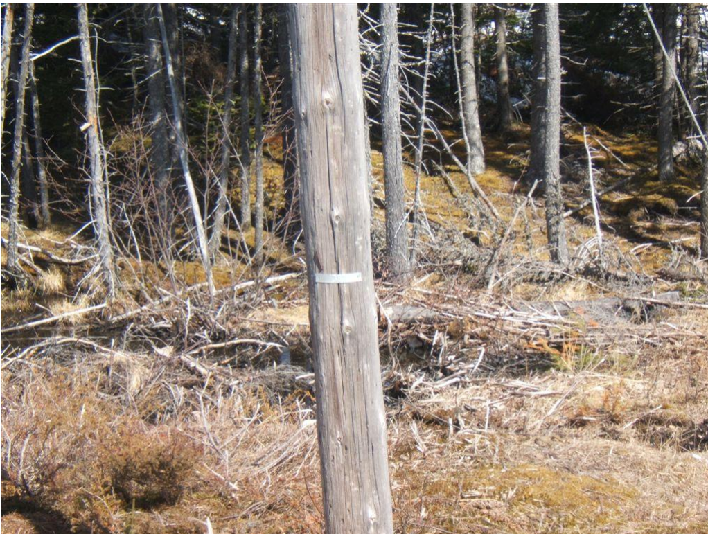
Figure 2 – 110L – Checks in pole
