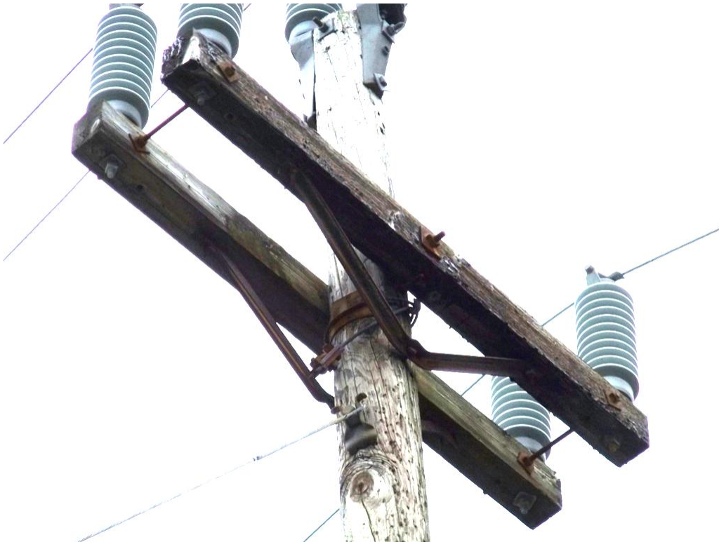
Figure 8 – 12L – Deteriorated crossarms
