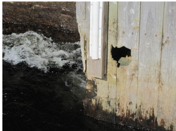
Figure 8 – Deteriorated Wood Structure
