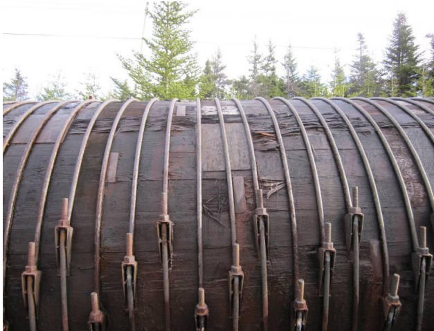
Figure 3 - Leak Repairs and Split Timbers
