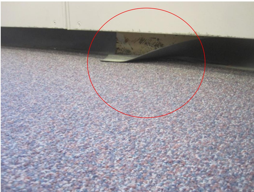
Figure 4 –Baseboards Losing Adhesion
