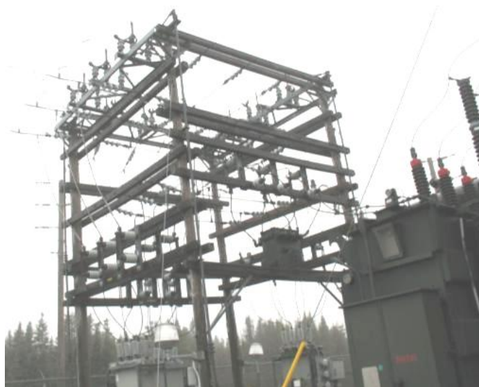
12.5 kV Wooden Structures & Bus
