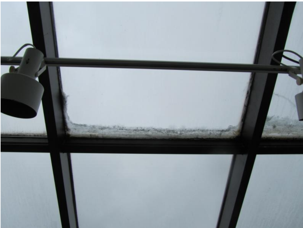
Figure 4 – Mildew on Atrium Roof Glass
