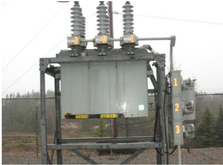
Hydraulic Recloser on TWG-03 Feeder
