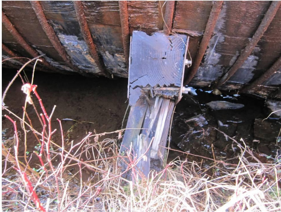
Figure 1: Typical Penstock Support Cradle Deterioration.
