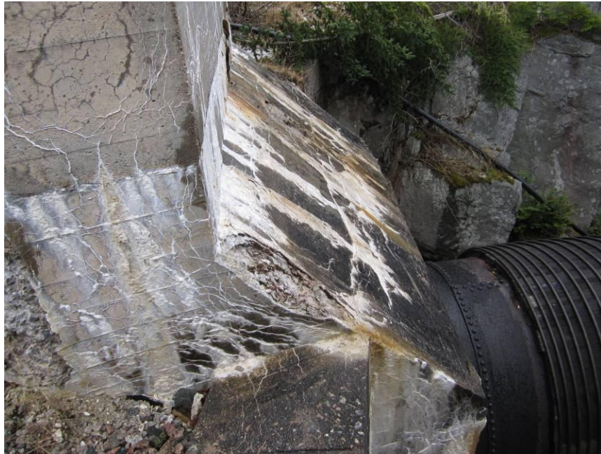
Figure 15: Intake Concrete Deterioration
