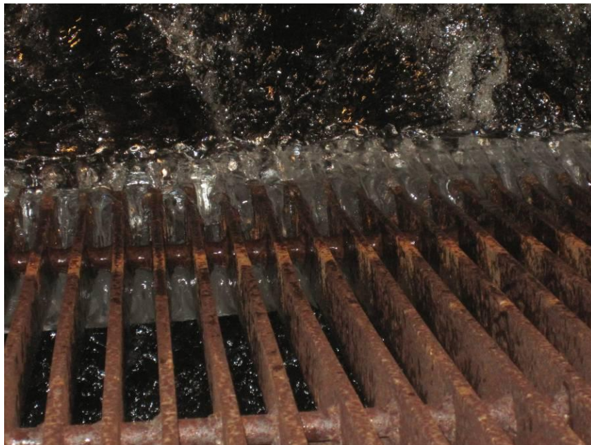
Figure 18: Ice Build-up on Trash Racks
