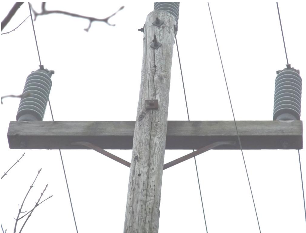
Figure 5 – 12L - Pole showing checking around bolts
