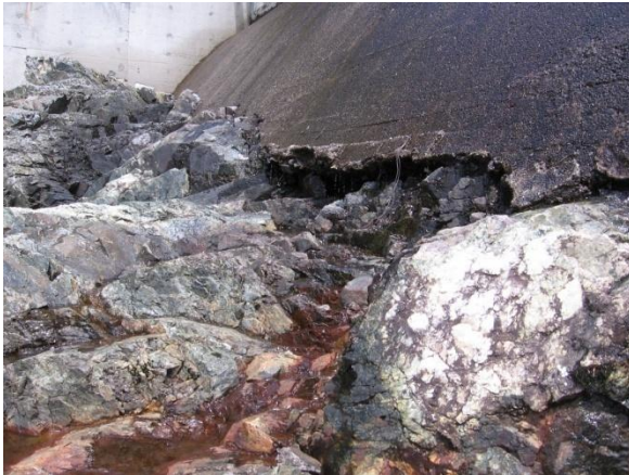
Figure 1 – Concrete Erosion at Spillway Toe
