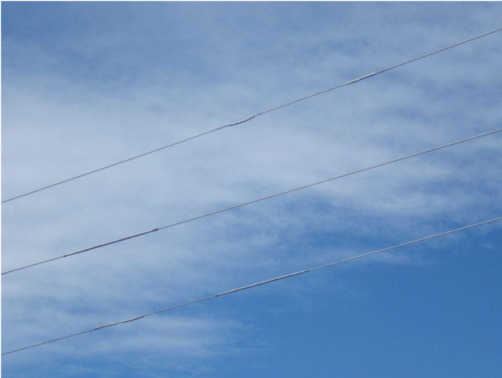
Figure 1 – 110L – Multiple sleeves to repair conductor damage
