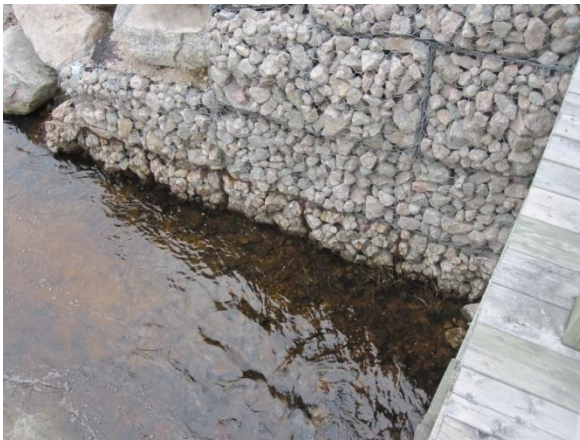
Figure 14 – Corroded Gabions - Downstream
