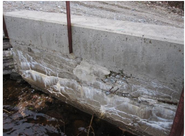
Figure 4 – Deteriorated Concrete on Upstream Face
