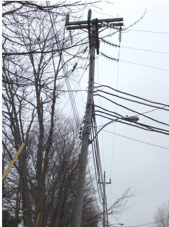
Figure 7 – 12L – Pole bent due to significant loading
