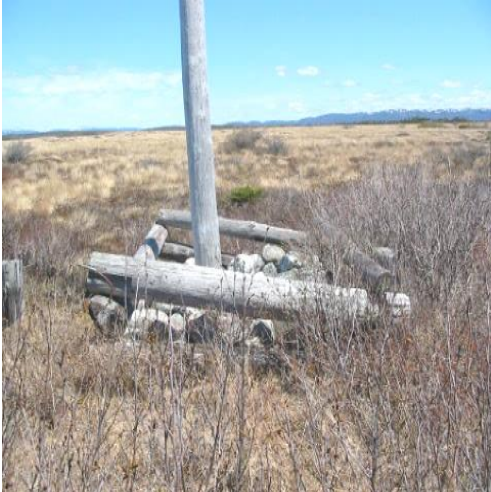
Figure 3: Pole Crib Requiring Repairs
