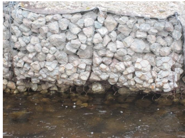
Figure 15 – Corroded Gabions - Downstream
