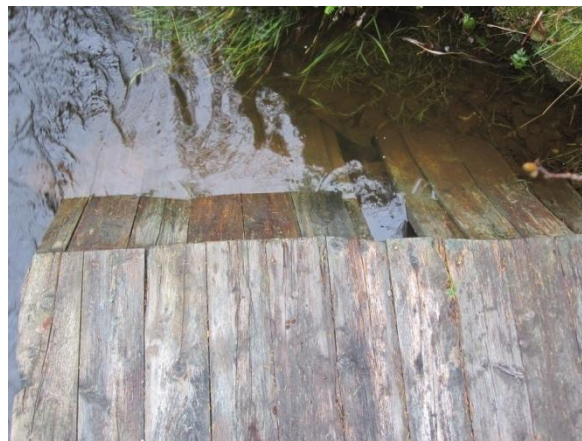
Figure 11 – Timber Deterioration
