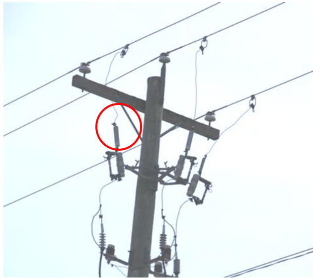
Figure 8: Current Limiting Fuses In Service
