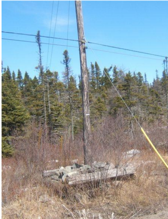
Figure 3 – 110L – Deteriorated pole and crib
