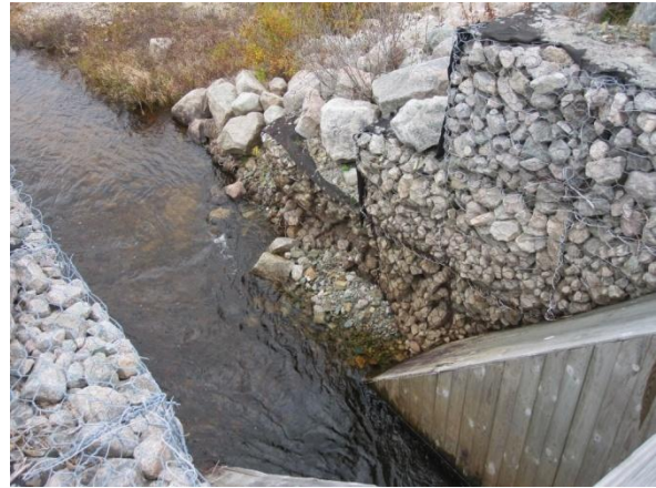
Figure 13 – Corroded Gabions - Upstream
