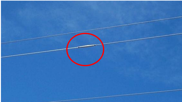
Figure 9: Automatic Sleeve In Service
