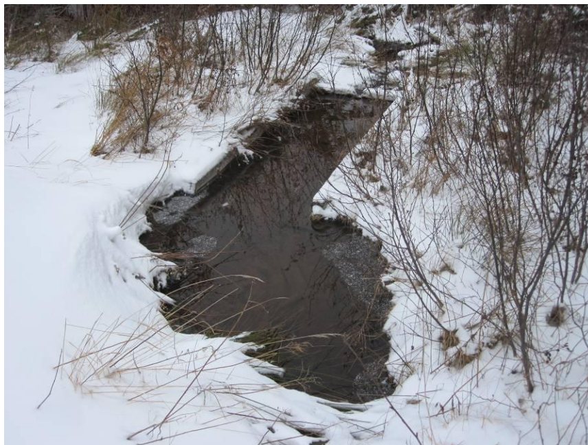
Figure 20: Leak under West Abutment
