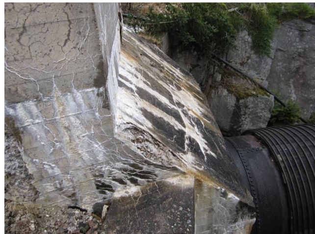
Figure 4 - Deteriorated Intake Concrete
