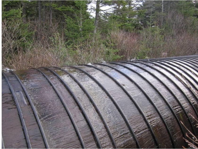
Figure 7: Leaking Joints along Length
