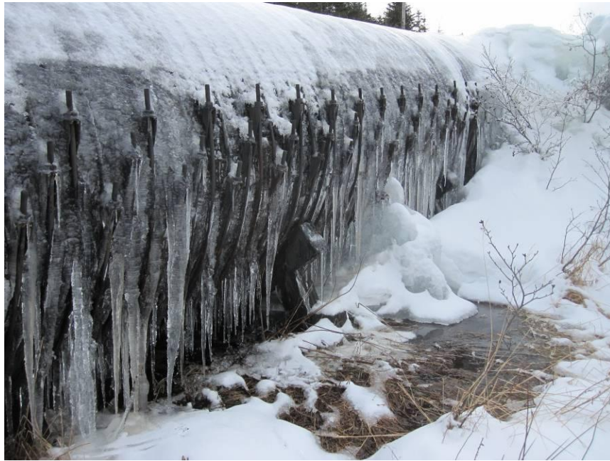
Figure 11: Ice Build-up on Penstock
