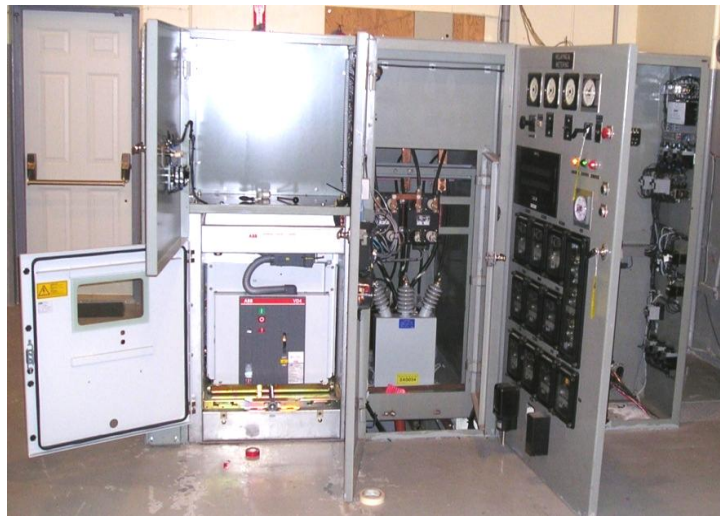
Figure 2 - Switchgear and Control Panel (doors open)
