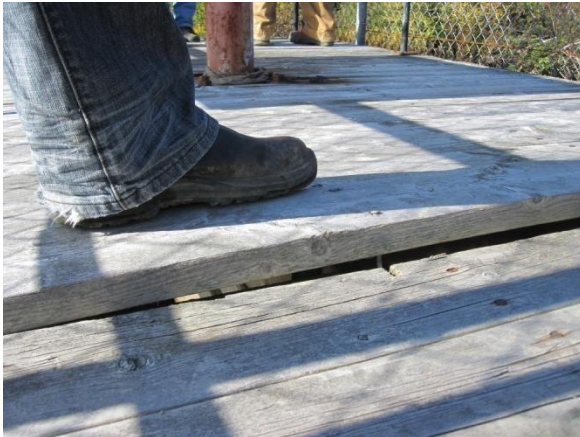
Figure 5 – Results of Settling Foundation
