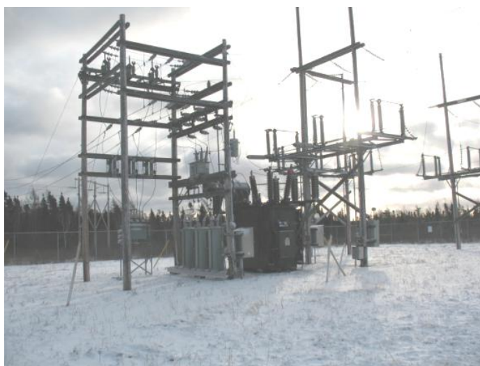
138kV & 25 kV Wooden Structures & Bus
