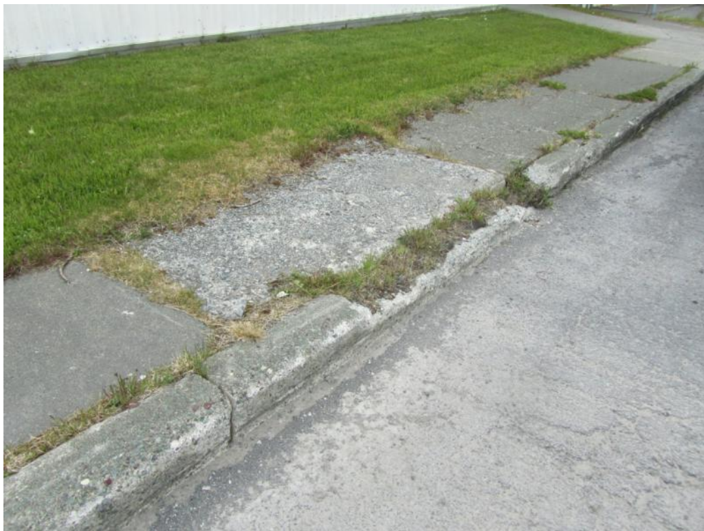
Figure 8 – Deteriorated Concrete Walkway
