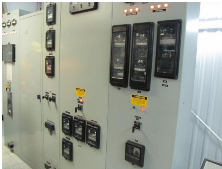
Transmission Line Electromechanical Relays
