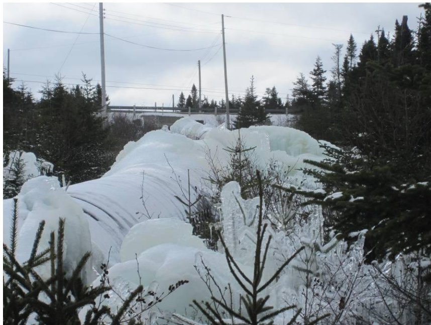
Figure 12: Ice Build-up on Penstock
