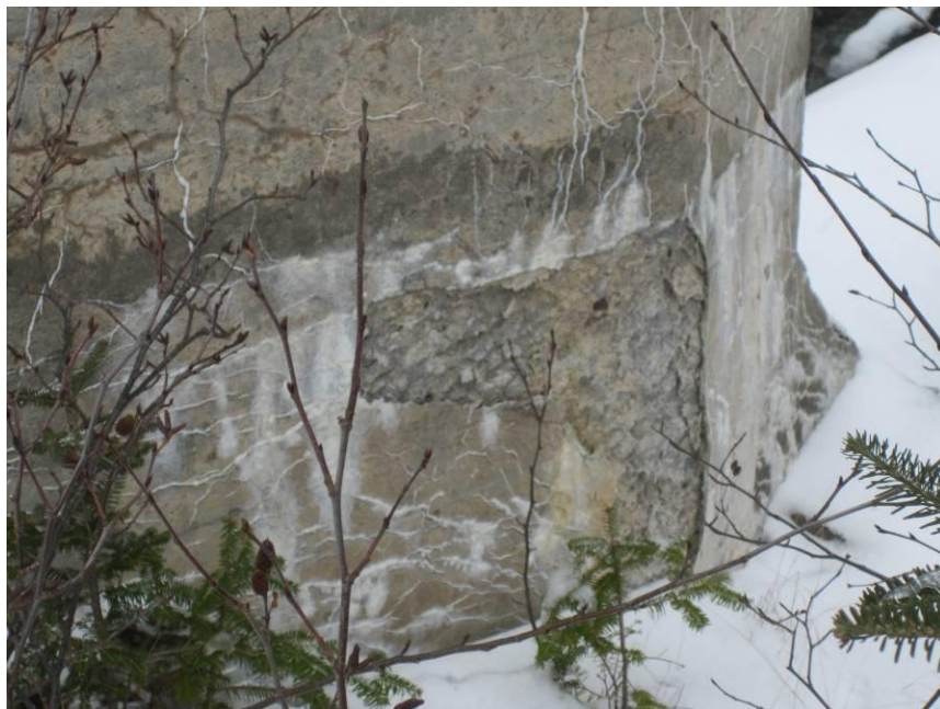
Figure 16: Intake Concrete Deterioration
