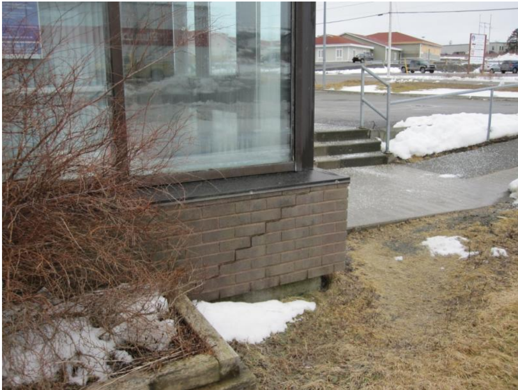
Figure 2 – Cracked Exterior Brick on Atrium
