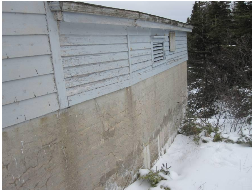
Figure 17: Deteriorated Building Envelope
