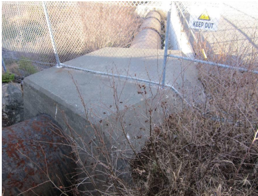
Figure 13: Steel Section (Note: Deteriorated Coating)
