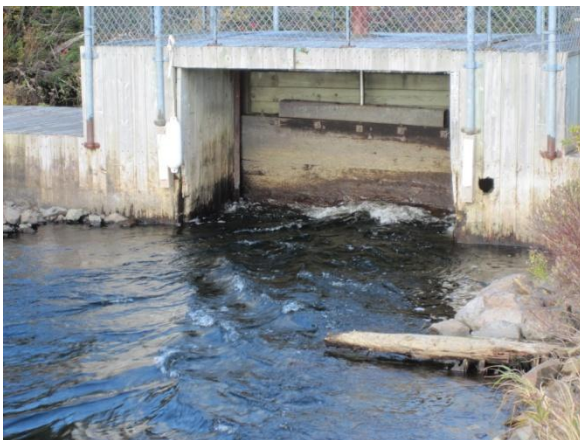
Figure 7 – Deteriorated Wood and Misaligned Gate
