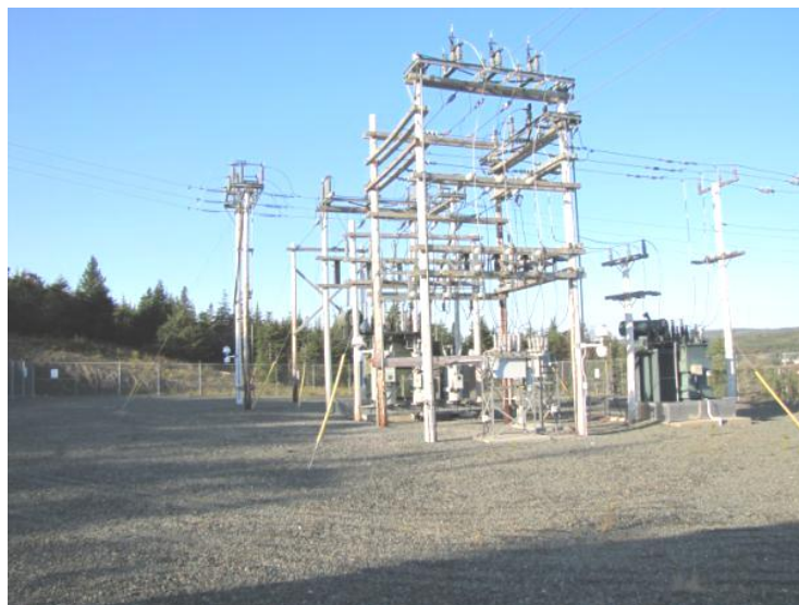
66 kV & 15 kV Wood Pole Structures and Bus
