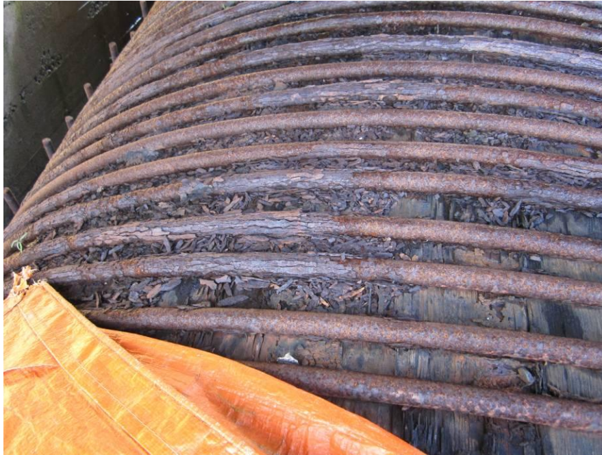
Figure 3: Heavily Corroded Steel Bands
