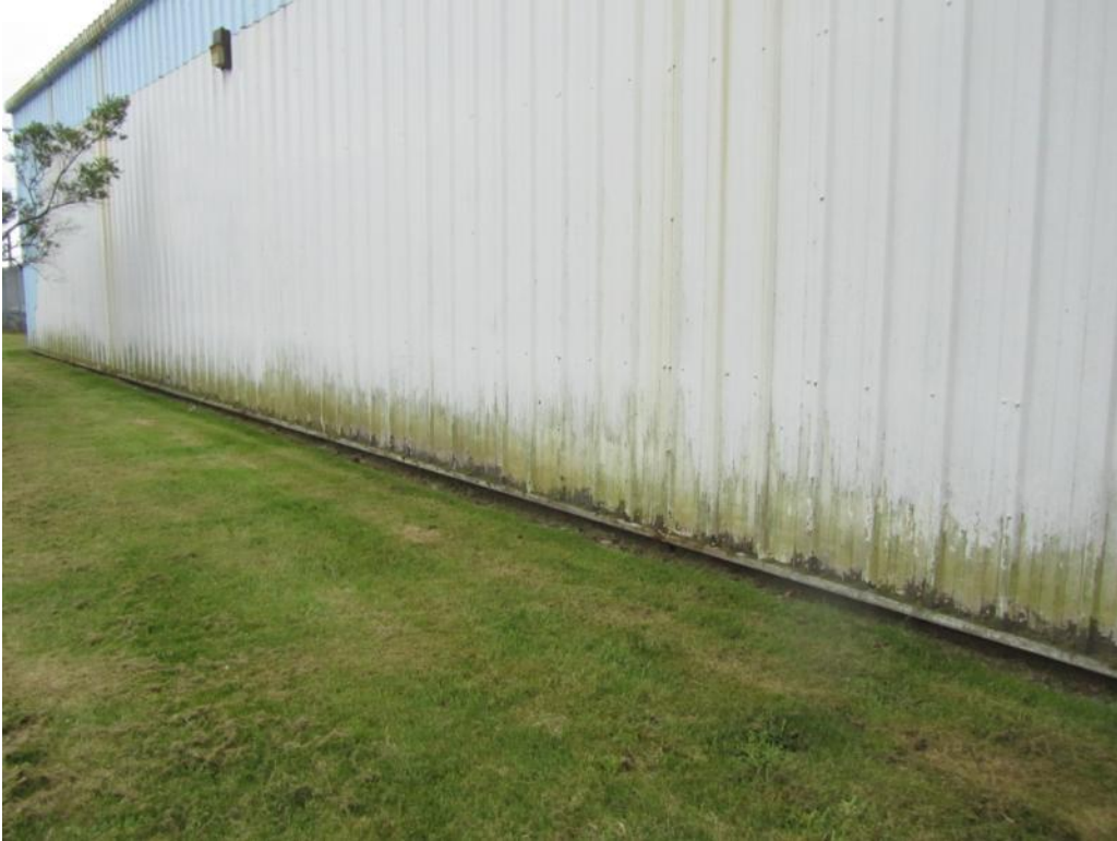
Figure 7 – Corrosion and Mildew on Exterior Siding
