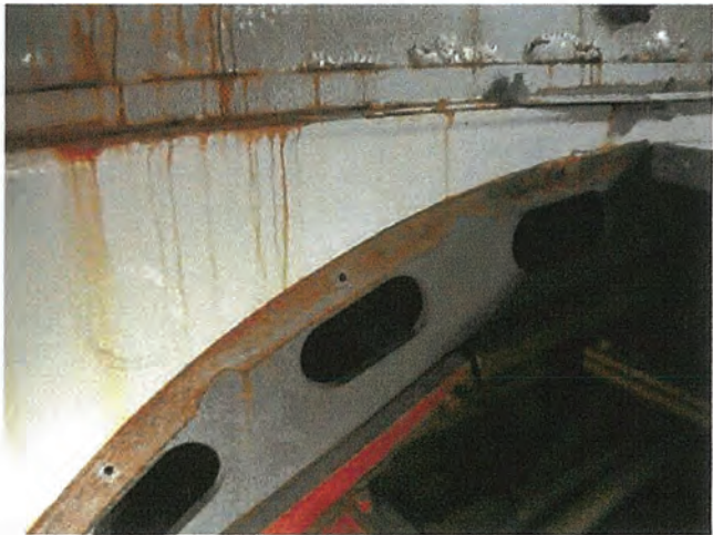
Roof top exhaust/ventilation is showing signs of corrosion and moisture ingress.
