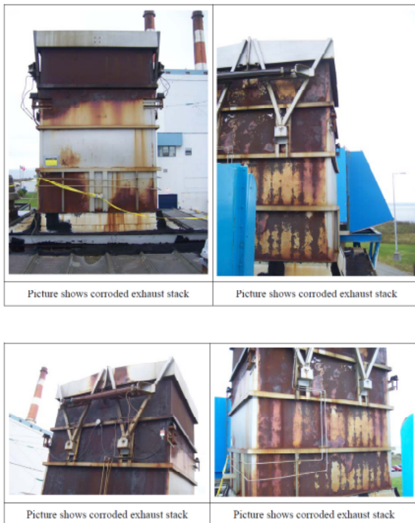
FIGURE 2-7 CORRODED EXHAUST STACK (GAS TURBINE PLANT)
