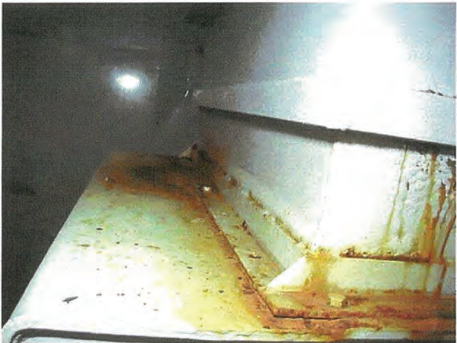
Roof top exhaust/ventilation paint flaking and corrosion.
