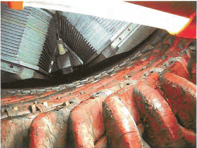
Connections between poles appear in good condition.
