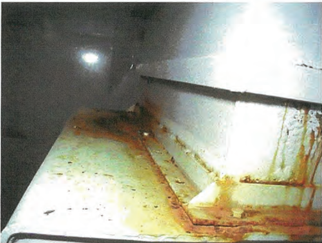
Roof top exhaust/ventilation paint flaking and corrosion.
