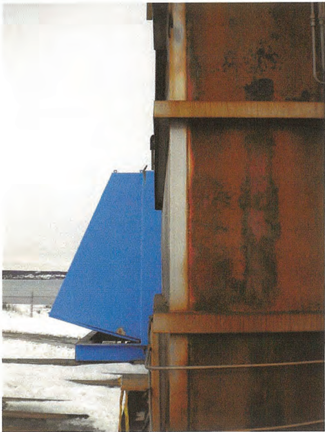
Figure 3 – Slight bulge in sidewall.
