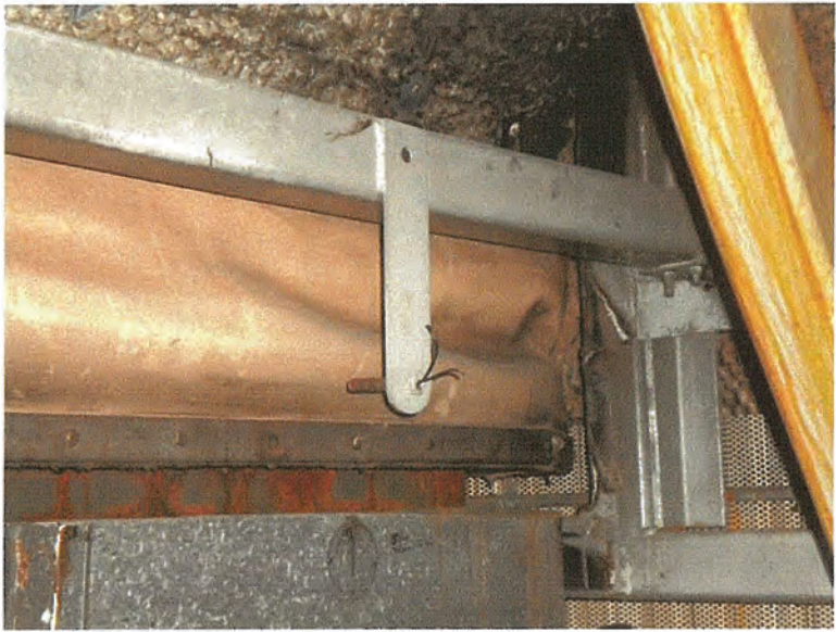
Figure 5 Expansion joint belt in good condition.
