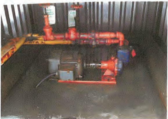
Both fuel oil pump (East and West) are in this enclosure
