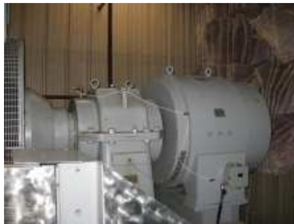
FIGURE 2-1 GTG GAS ENGINE & GENERATOR
