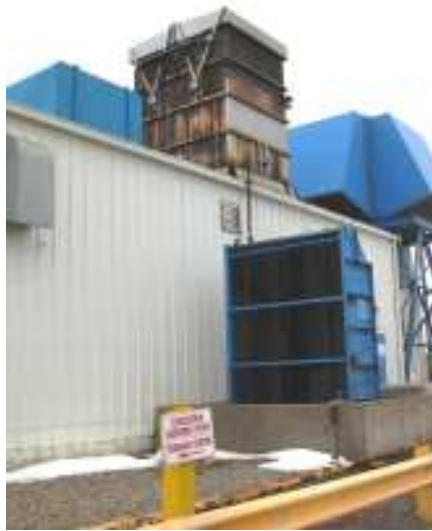
FIGURE 2-4 LIGHT OIL RECEIVING & LUBE OIL RADIATOR
