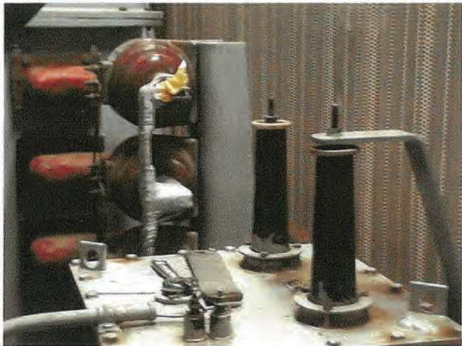
Star Point had to be disconnected from transformer for true reading. With this point connected insulation resistance to ground reading is 2000 Ω.
