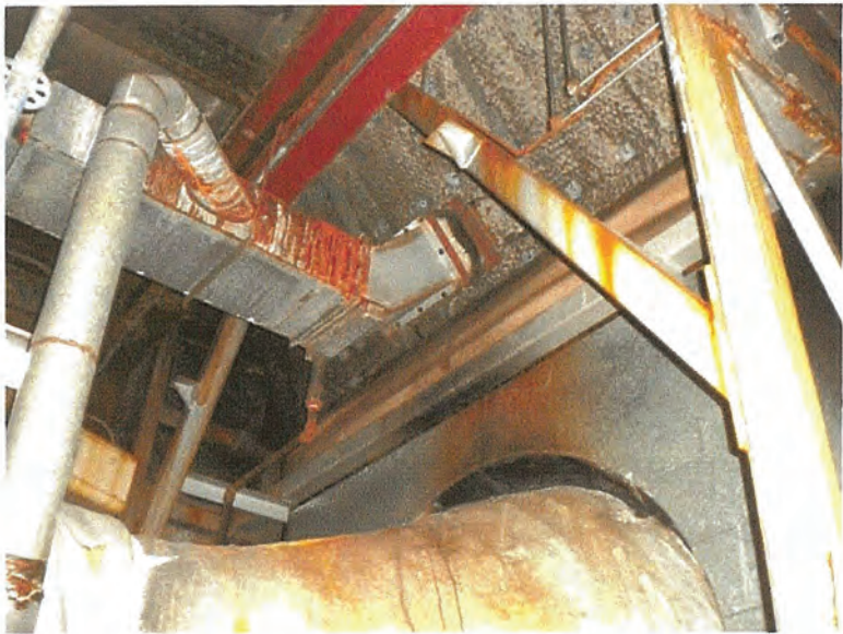
Figure 4 Transition area of with external insulation above the exhaust plenum.
