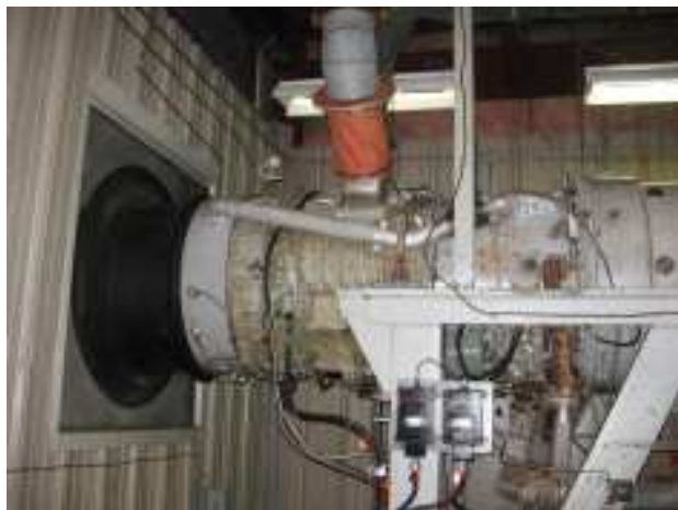
FIGURE 2-1 GTG GAS ENGINE & GENERATOR
