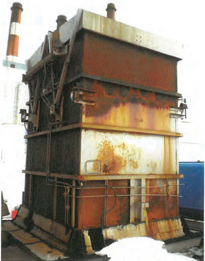
evidence of no or minimum amount of internal insulation.
