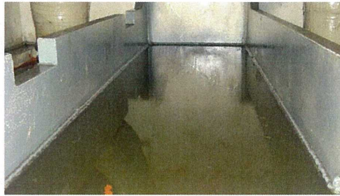
Bushing Box – Oil and Water in bottom
