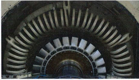
View of CE End Windings with unit on Half Joint
