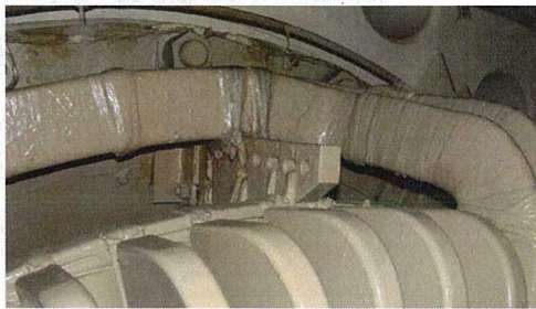
CE End Winding Greasing
