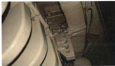
CE End Winding Greasing
