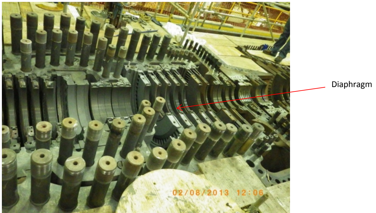
Figure 2. Steam Turbine HP Bottom Casing with Rotor Removed
