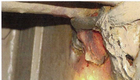
CE End Windings Greasing
