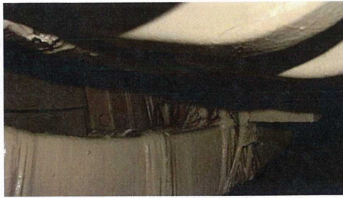
CE End Winding Greasing
