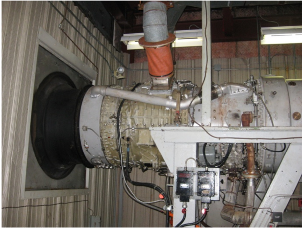
FIGURE 11-36 GTG GAS ENGINE & GENERATOR
