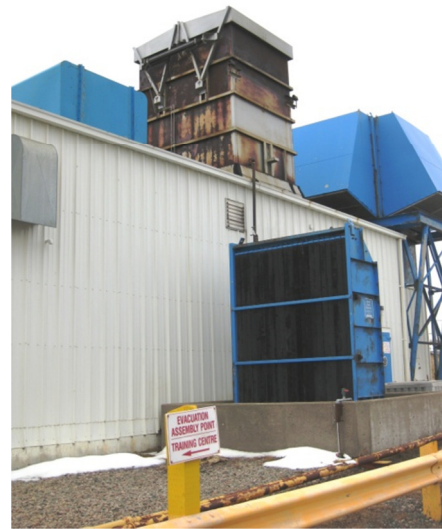
FIGURE 11-35 LIGHT OIL RECEIVING & LUBE OIL RADIATOR
