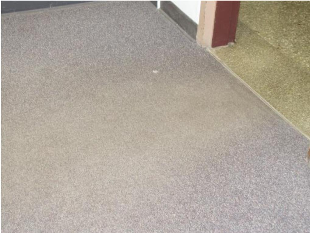
Figure 8 - Deteriorated carpet in high traffic area
