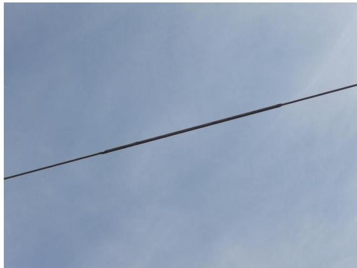
**Figure 16 – Armour Rod to Repair Wire Damage 124L**
