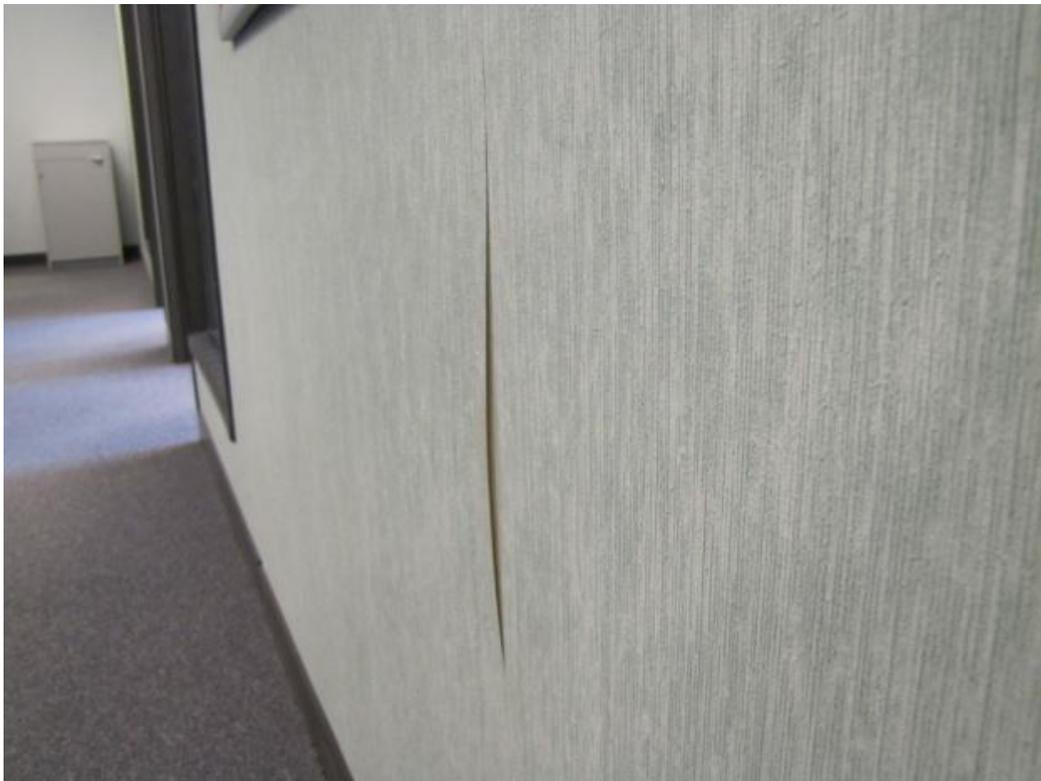
Figure 11 - Wall covering losing adhesion
