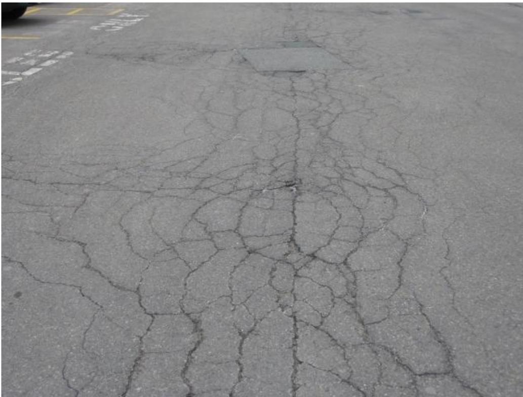
Figure 4 -Spider cracking west end of parking lot
