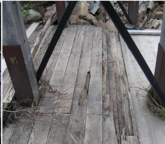
**Figure 2 - Long Pond Dam (Deteriorated Decking)**
