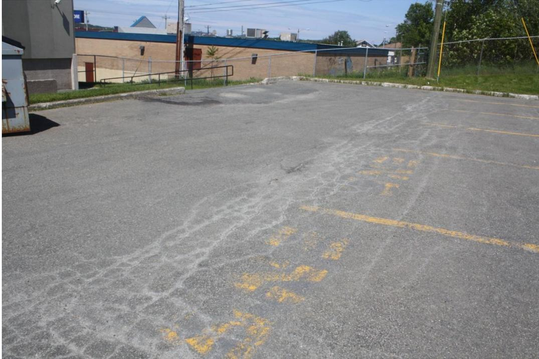
Figure 5 – Spider cracking east end of parking lot
