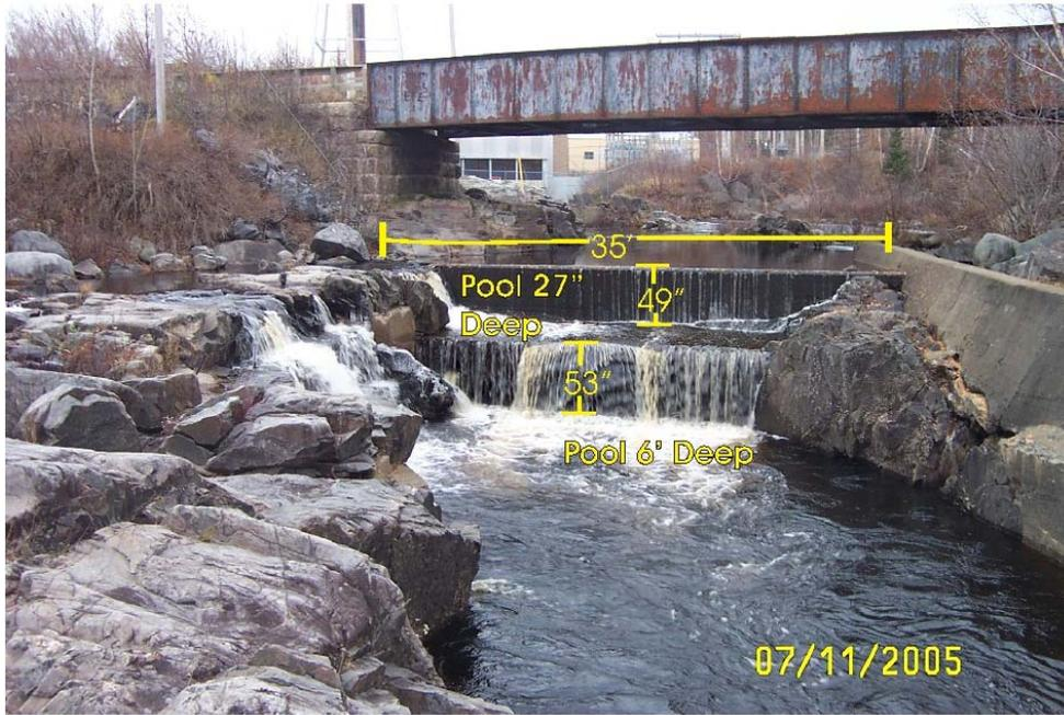
Figure 3 - Dimensions of Tailrace obstacle
