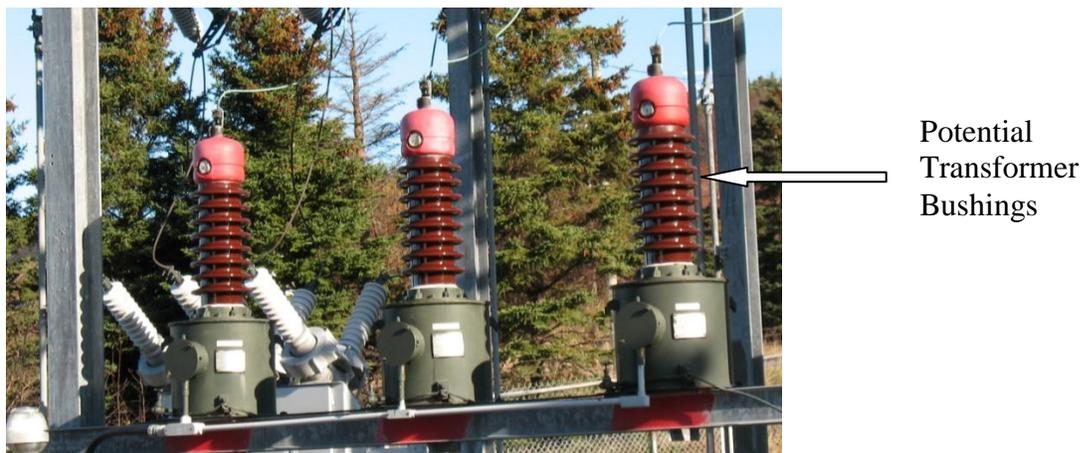
Figure 3 - 66 kV Potential Transformers
