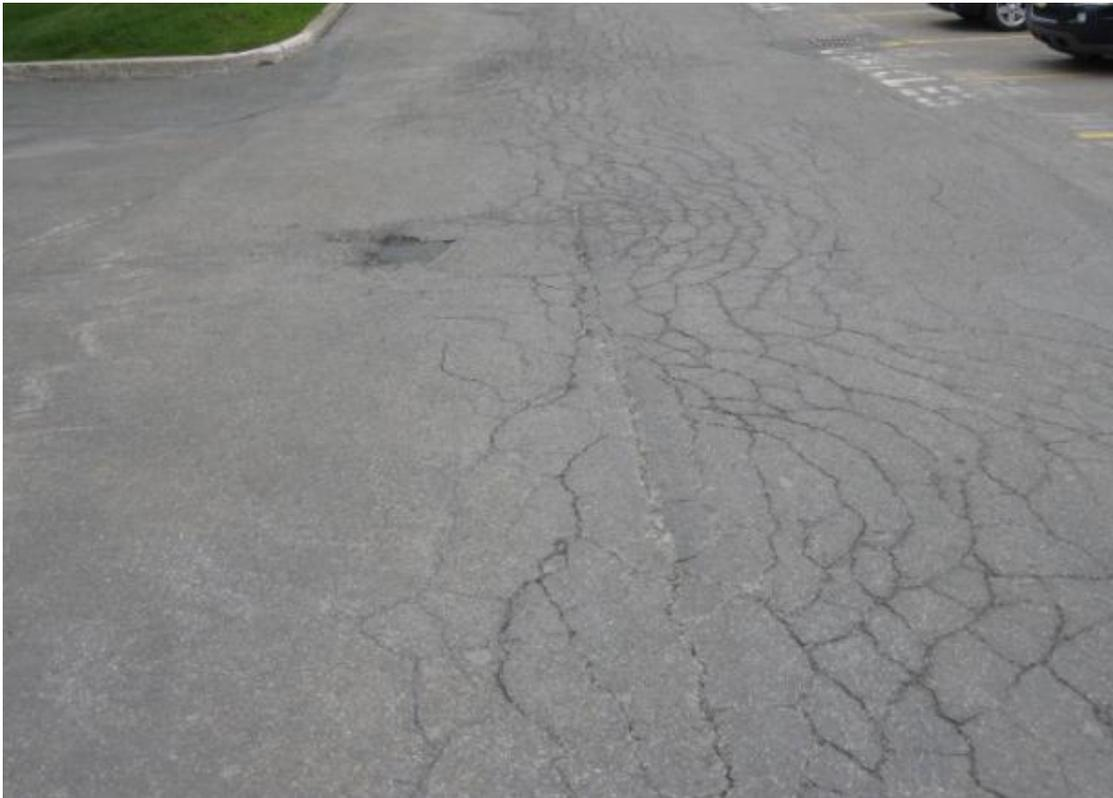
Figure 1 - Spider cracking center of parking lot
