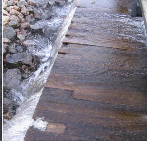
Figure 7 - Delaminating Spillway Decking
