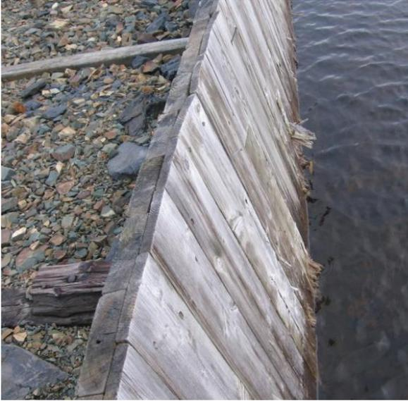
Figure 6 - Misaligned Timber Facing with Ice Damage
