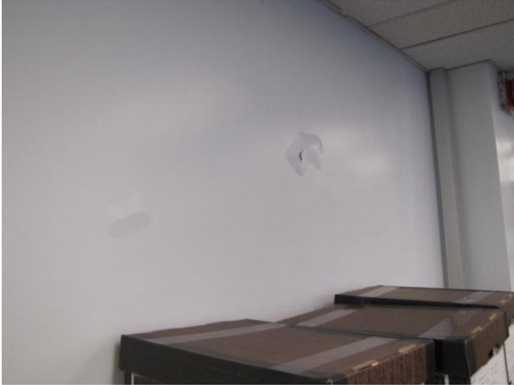
Figure - 10 Paint peeling from concrete block wall
