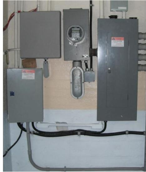
**Figure 4 – AC Panels & Meter**
