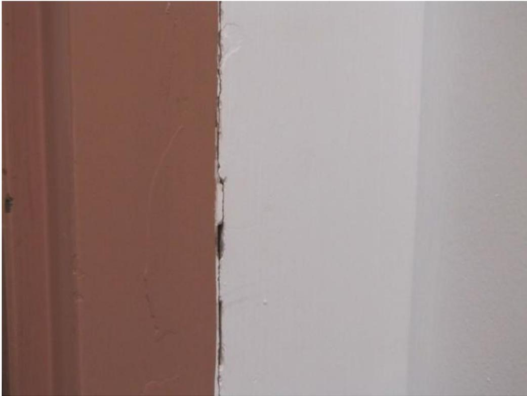
Figure 12 - Plaster cracking around door frame
