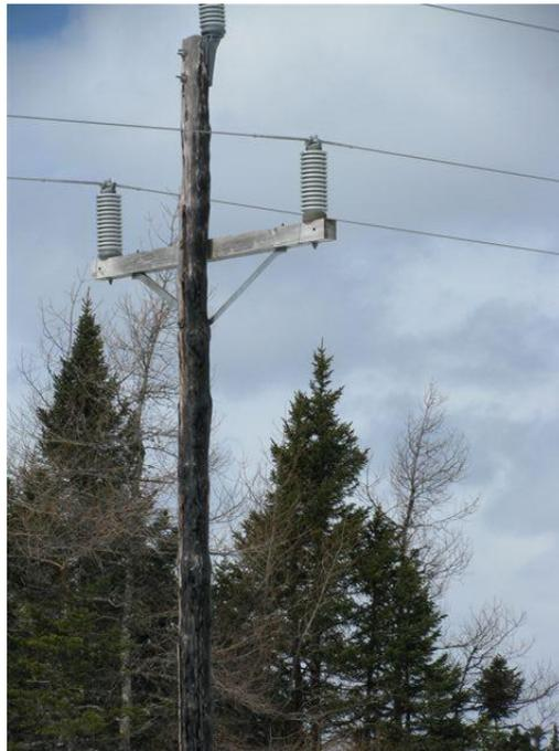
**Figure 2 – Deteriorated Pole on 110L**
