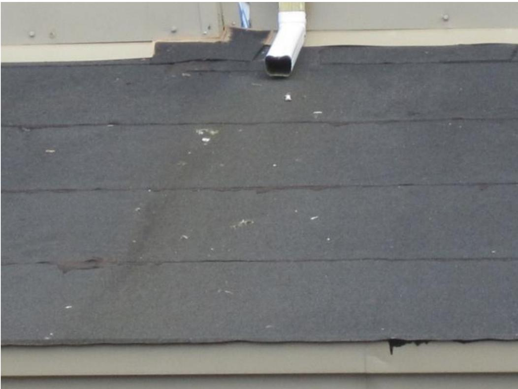
Figure 15 – EMC Deteriorated Roof
