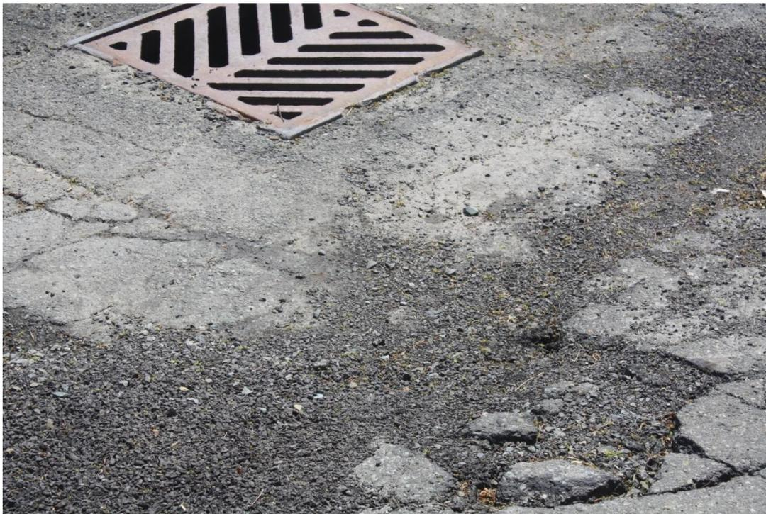
Figure 6 - Deteriorated asphalt near catch basin
