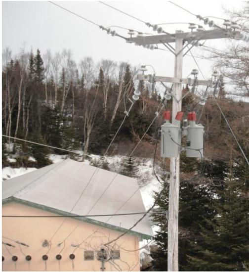
**Figure 3 – Station Service Transformers**
