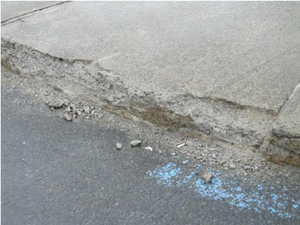
Figure 3 - Deteriorated curb
