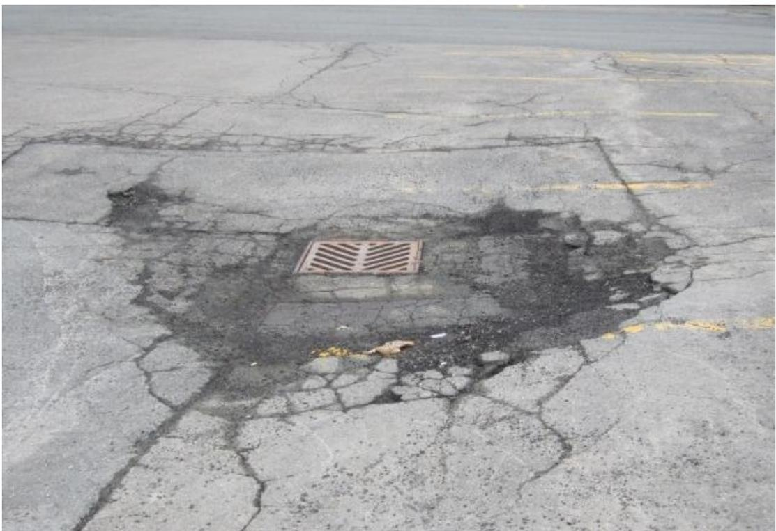
Figure 2 - Deteriorated asphalt and catch basin
