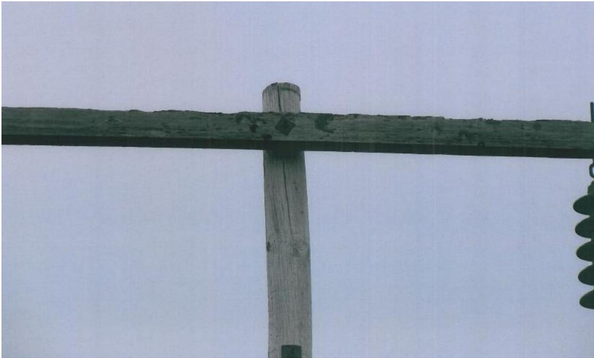
**Figure 13 – Deteriorated Pole and Crossarm 21L**
