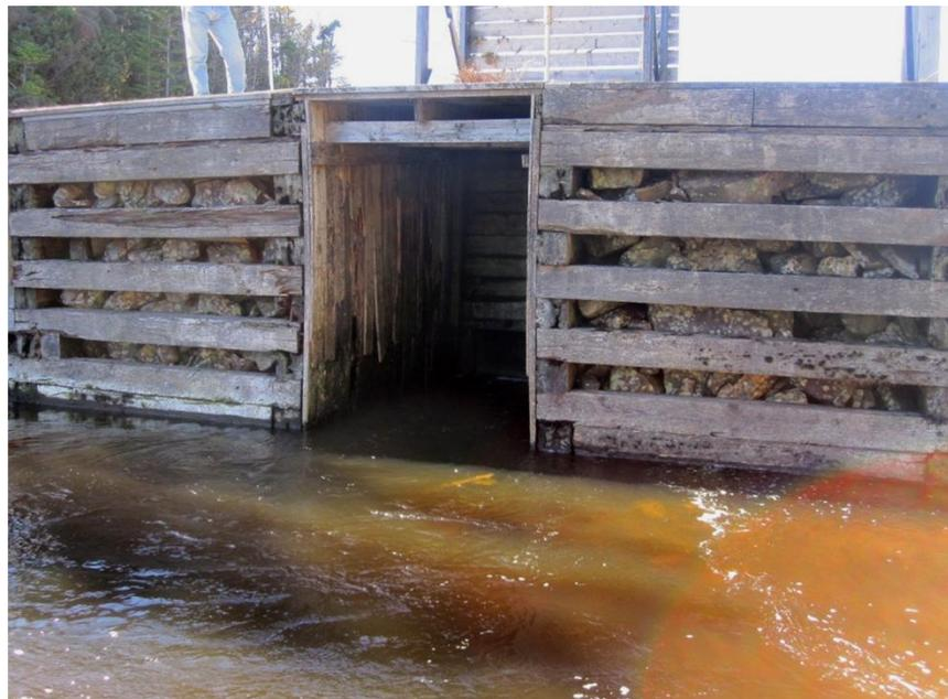
**Figure 3 - Long Pond Dam (Deteriorated Outlet and Cribbing)**
