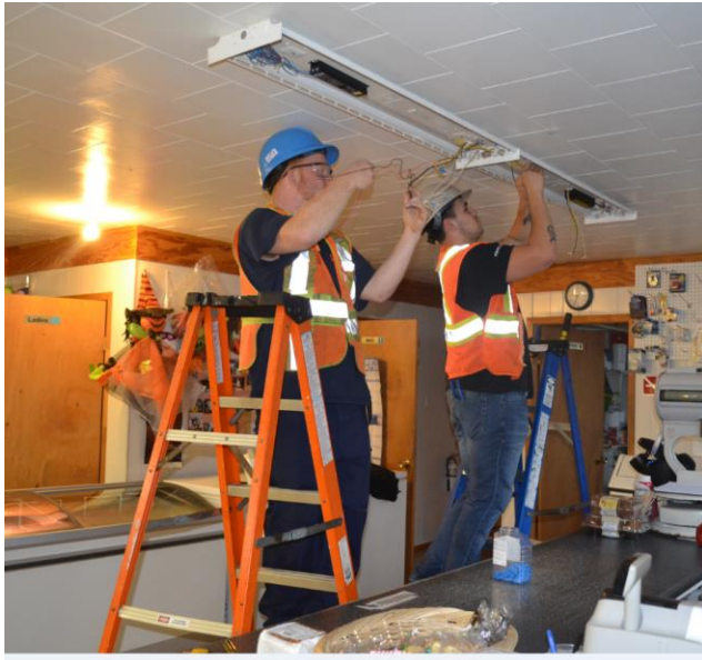
Powells Electrical team replacing T12 bulbs for T8 LED's in McCallum.
