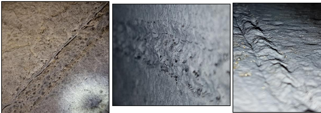
Figure 3-3: Longitudinal Seams in Penstock No.1 Section 16
